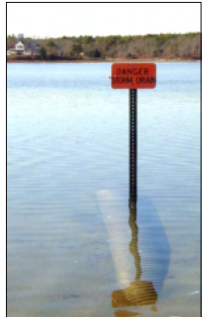
Figure 1. A submerged stormdrain in Wareham.
