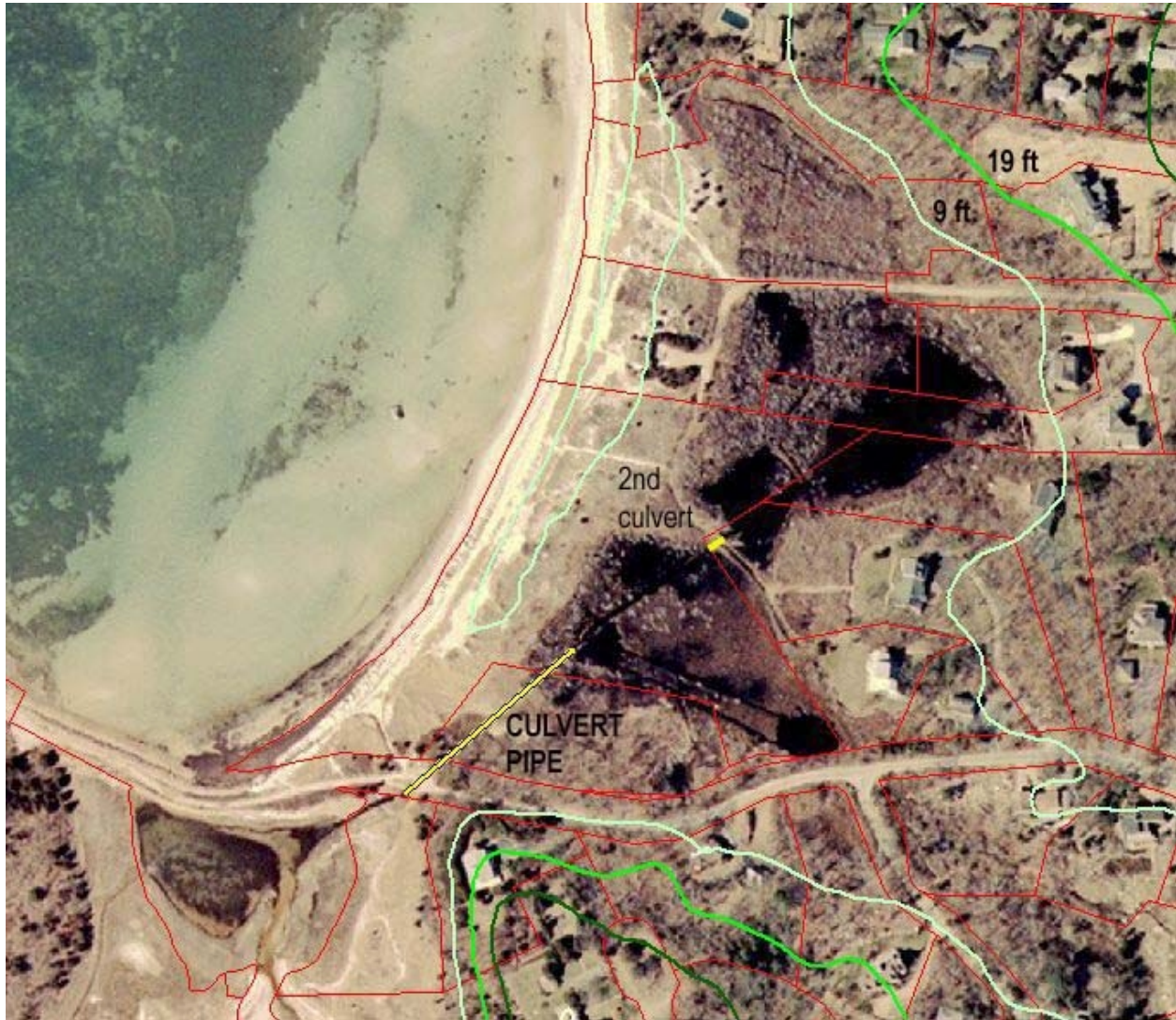
Figure 1. Existing culvert pipe, approximate property boundary (red lines), and topographic contours (light green = 9 feet, bright green = 19 feet) in the vicinity of Little Island Salt Marsh. Property bounds from Town of Falmouth. Contours from MassGIS based on photo interpretation.
