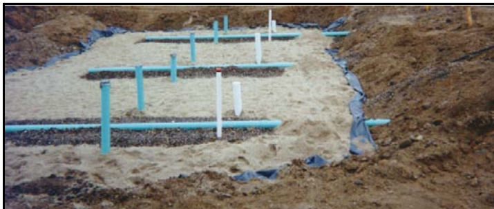
An SAS during construction. Each trench receives a fourth of the discharge from each test replicate. Dosage is 0.74 gallons per sq. ft. per day.
