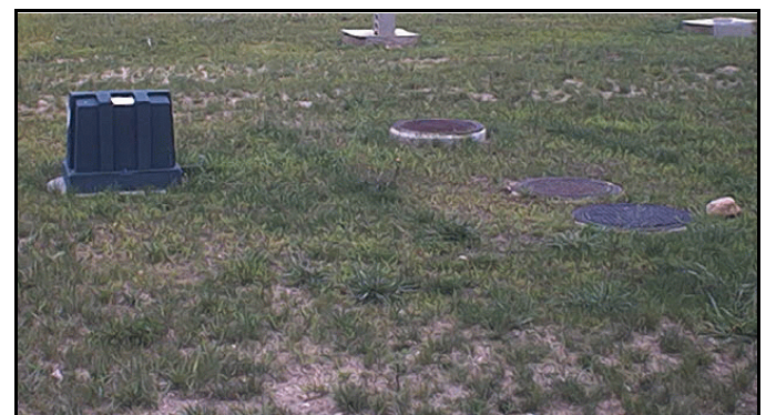
MicroFAST after installation.
