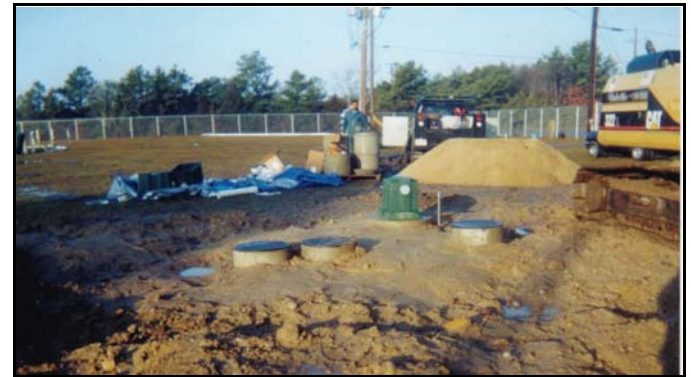
MicroFAST during construction.
