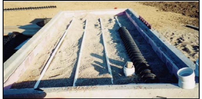
Sand Filter Bed during installation.
