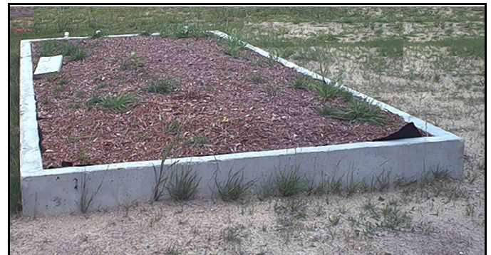
Sand filter bed after 6 months.
