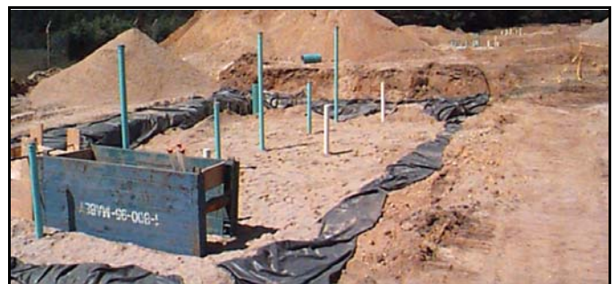
SAS trench with sampling wells at construction.
