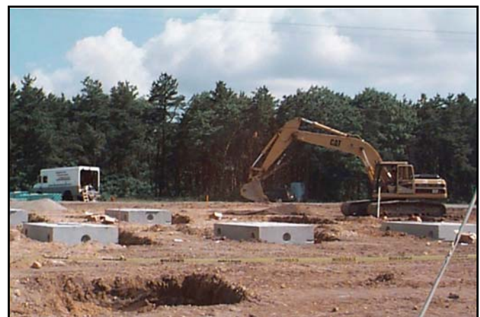
Septic tanks during installation.
