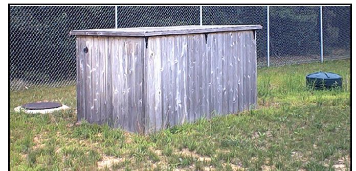
One unit, after installation.
