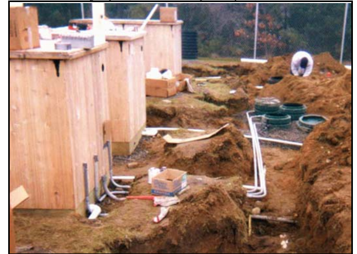
Waterloo Biofilter during installation (3 side by side installations)
