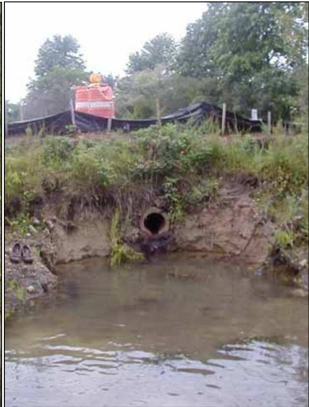
Figure 3. Same location as Figure 2 just three days later (8/16/04) after another moderate rainfall showing even greater erosion and the formation of a plunge pool.
