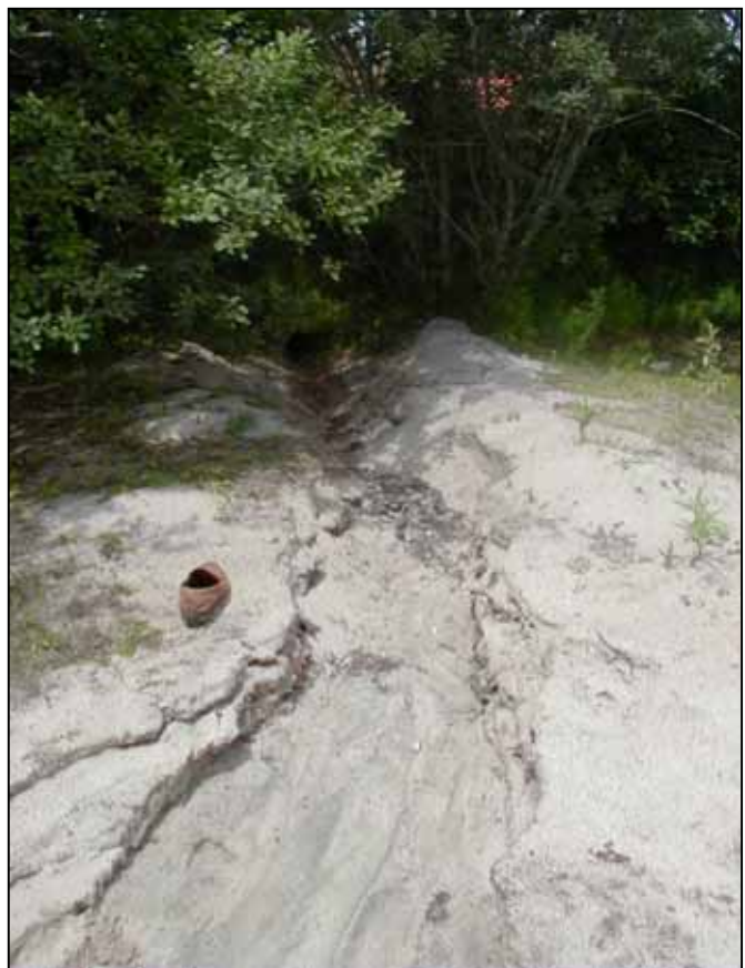
Figure 1. Gully in recently deposited sediments and old sediments of a delta in front of a discharge pipe in an area of the pond exposed due to low water levels (Photo taken 8/13/04 , Joe Costa) .
