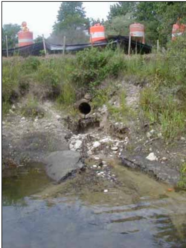
Figure 2. Bank erosion (at location B in figure 5), and gully in recently deposited sediments in another area of Sols Pond (Photo taken 8/13/04 , Joe Costa) .
