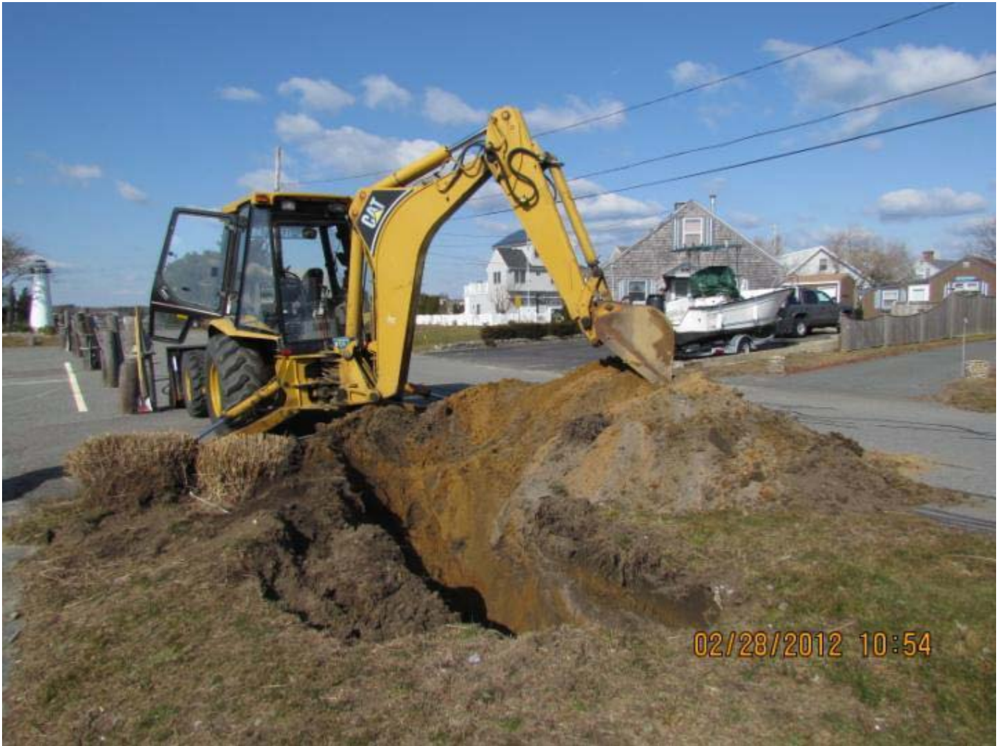
Figure 2: Soil pit #1 backhoe trench.
