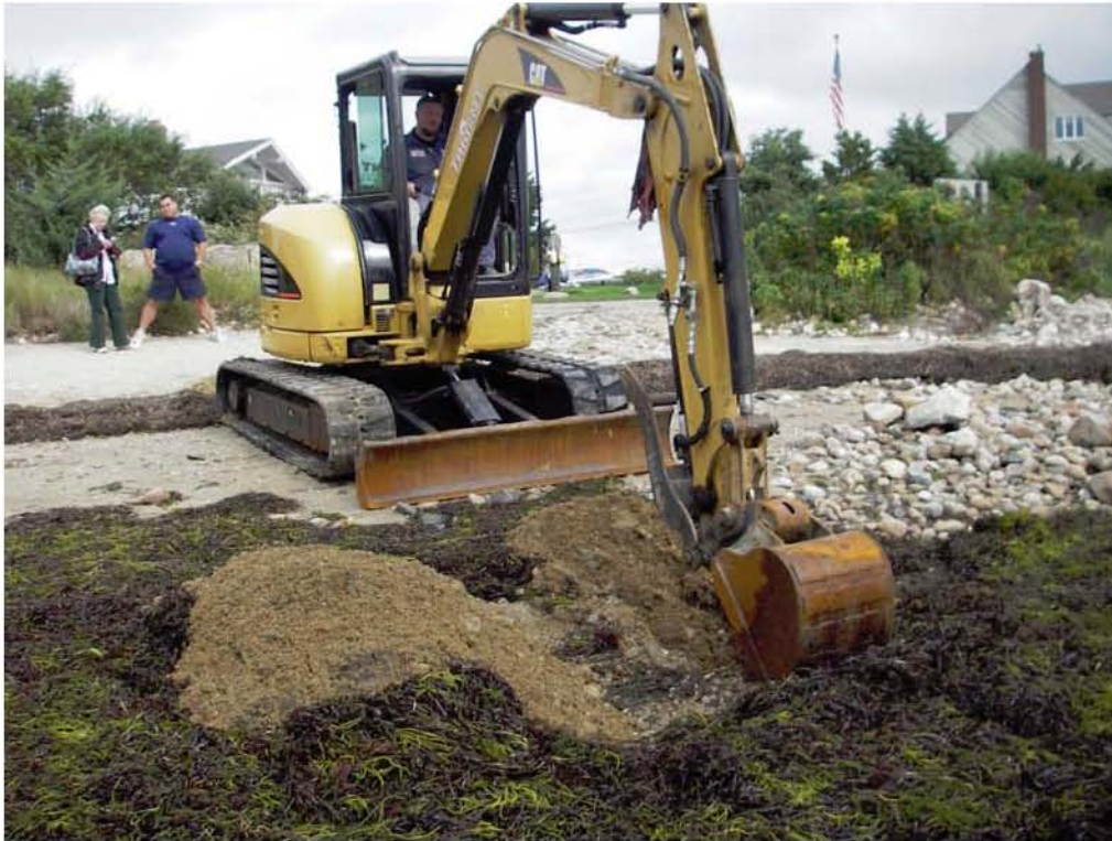
1. Test pit excavation in cobble shoreline at Leisure Shores.
