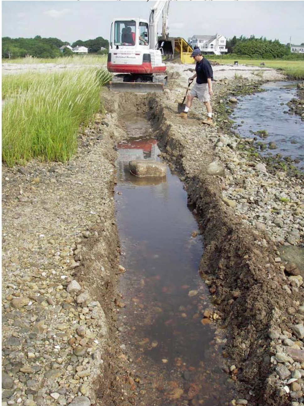
3. Trench/test pit excavation.
