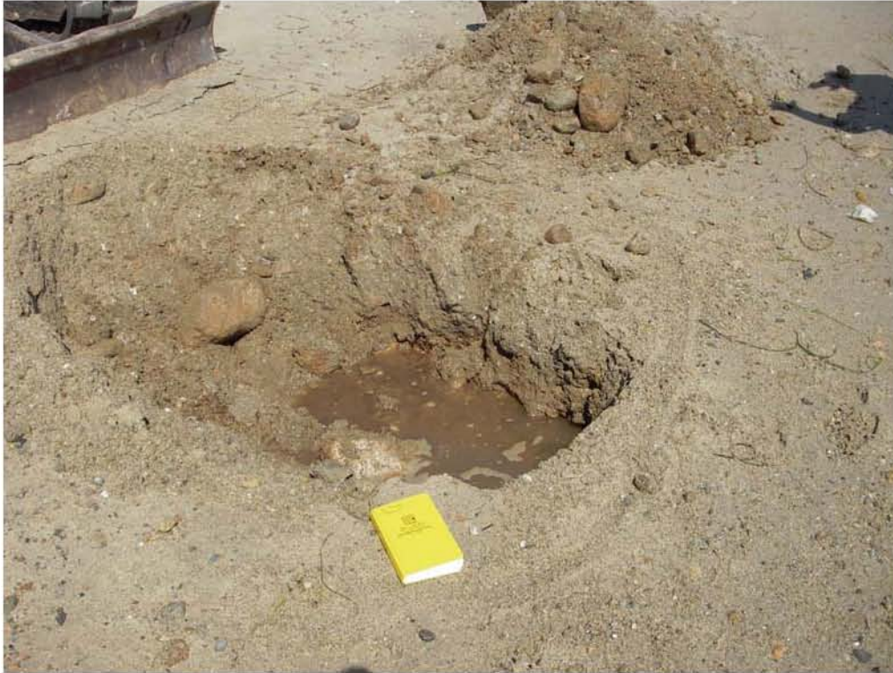
1. Test pit excavation at Leisure Shores.
