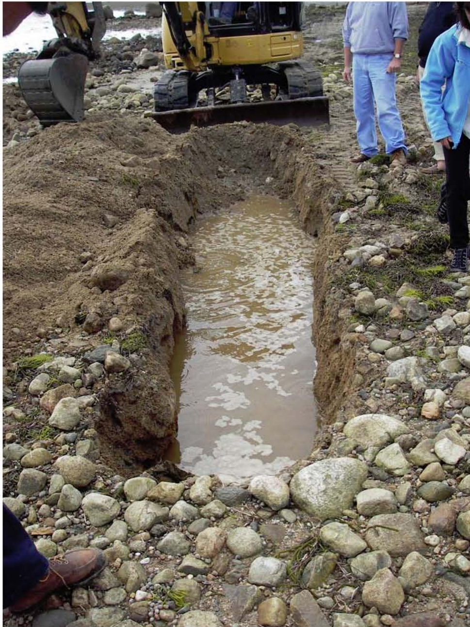
6. Test pit excavation (T093008.22)
