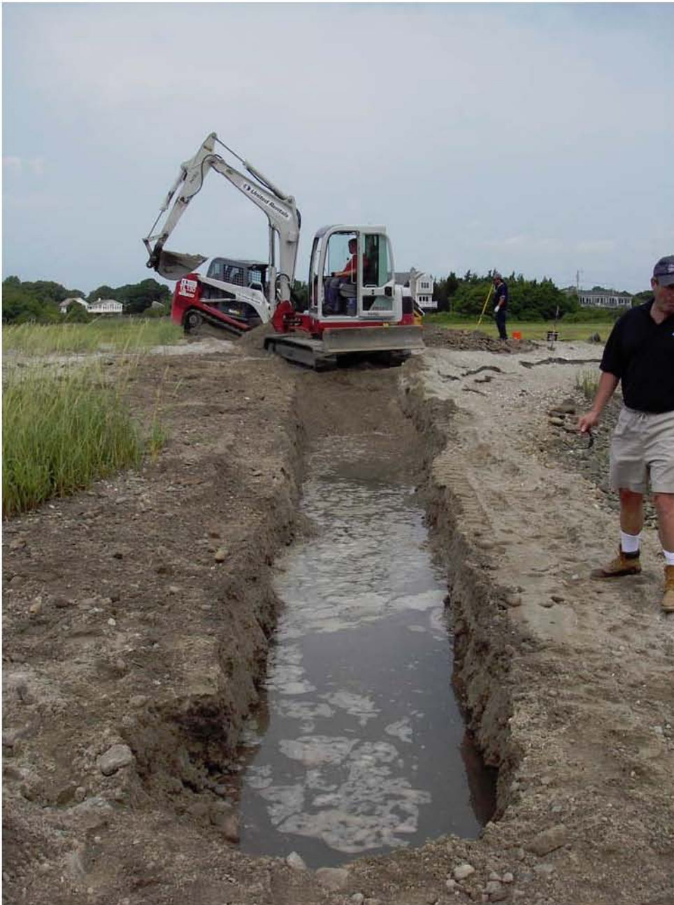
4. Trench/test pit excavation.
