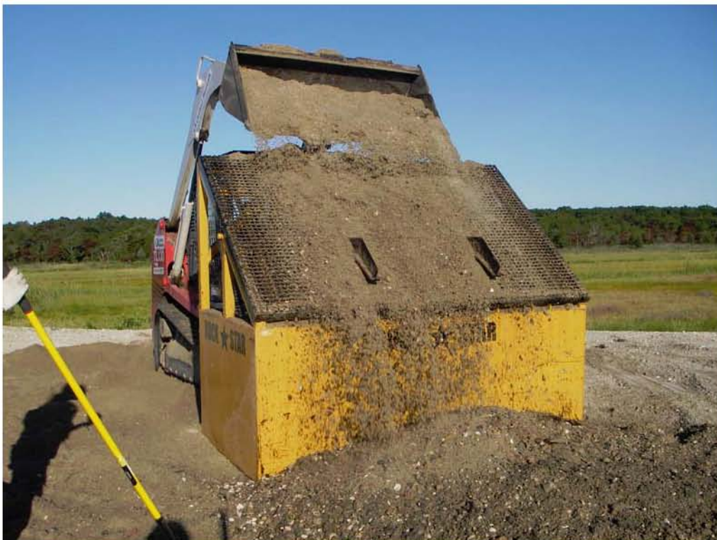
6. Screening excavated material.
