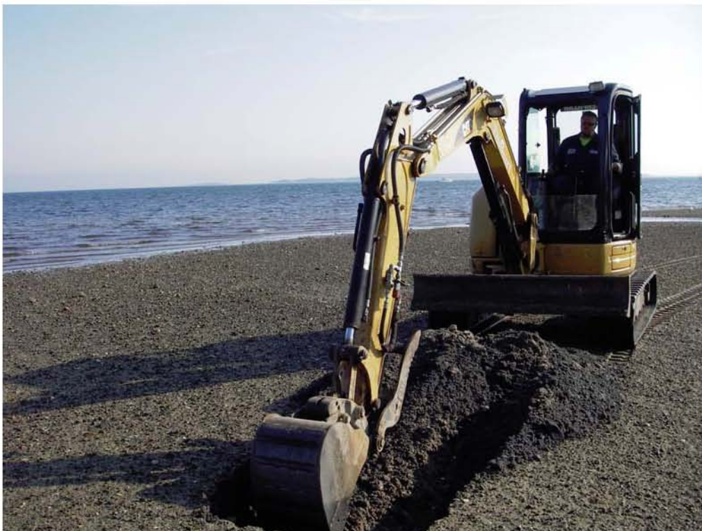
2. Test pit excavation.
