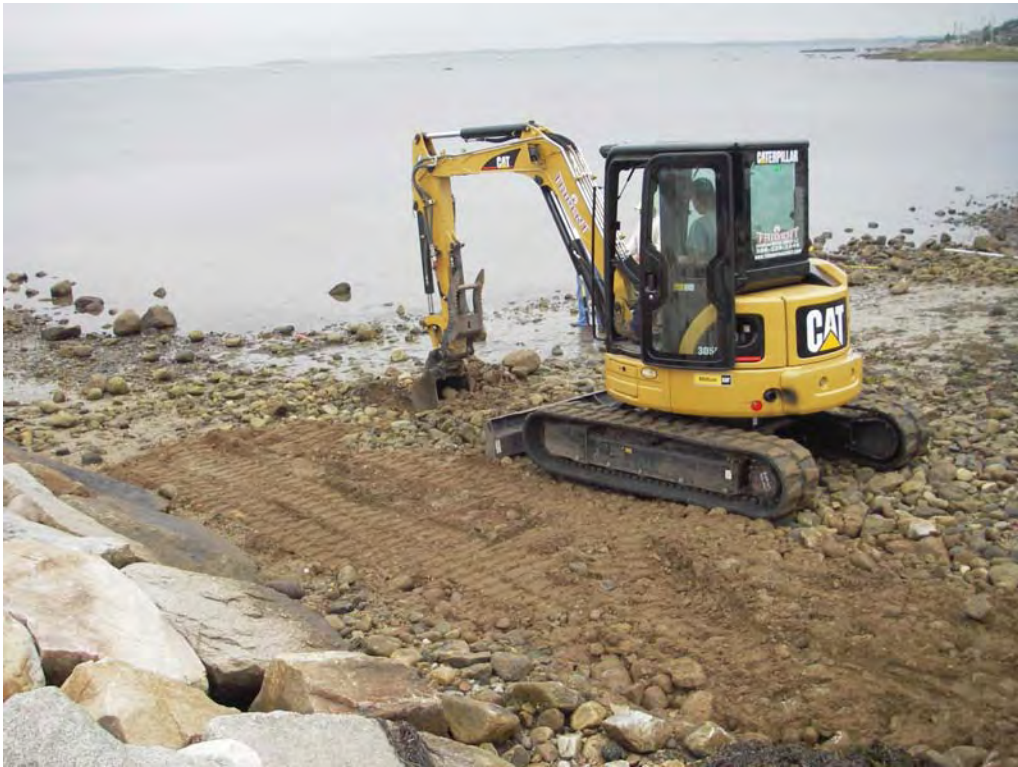
1. Trench excavation in cobble beach area – September 10, 2007.
