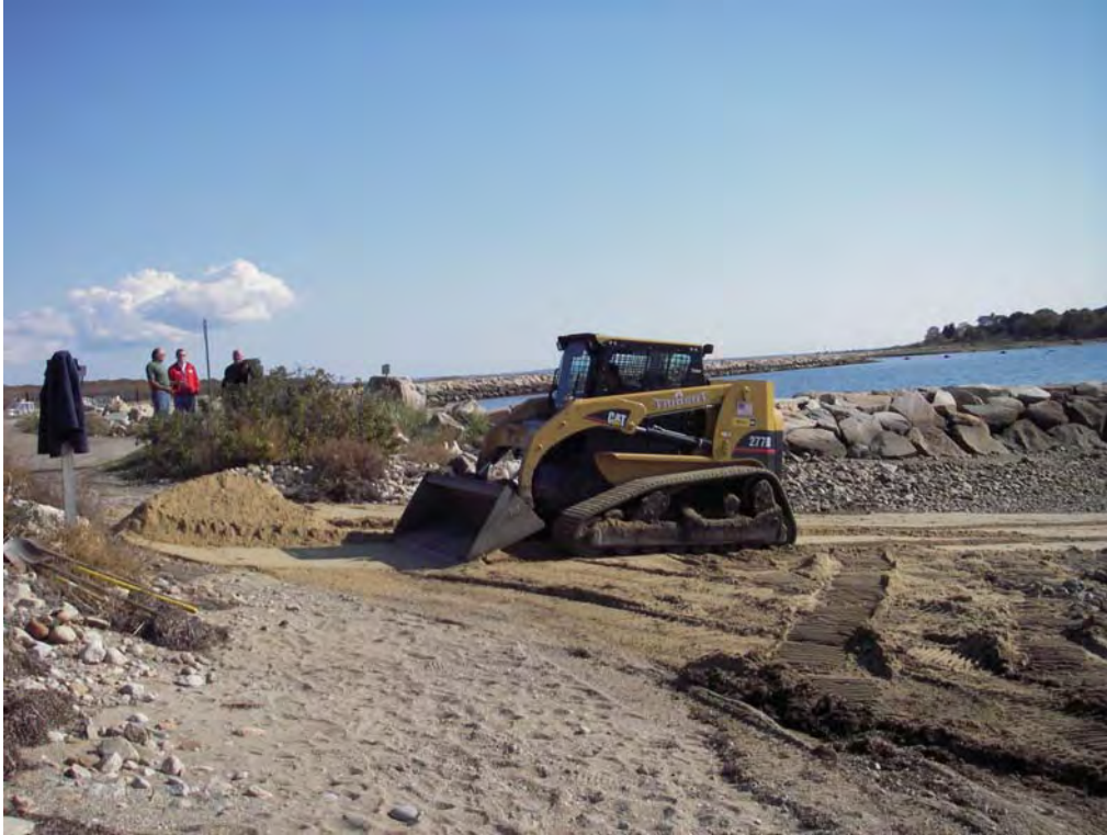
12. Sand replacement – November 5, 2007.
