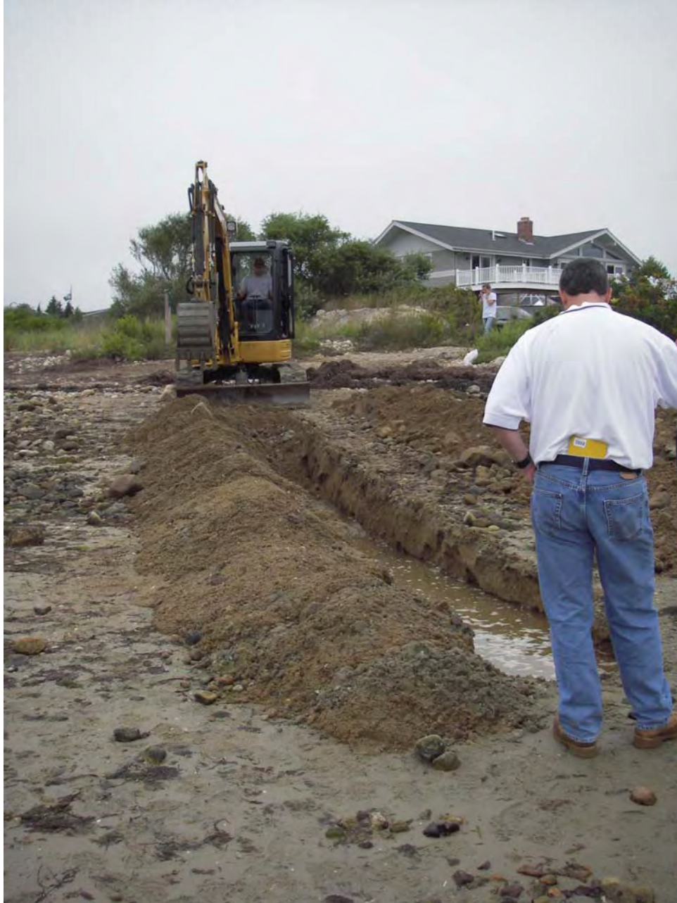
3. Trench excavation in cobble beach area – September 10, 2007.
