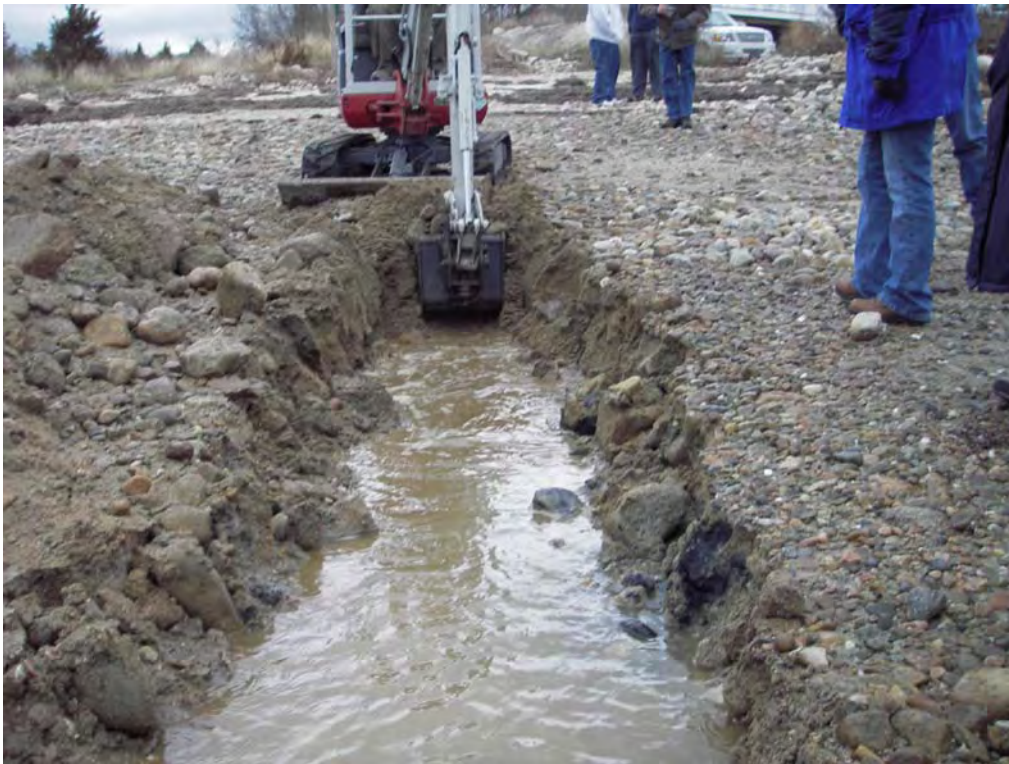
13. Trench excavation – December 7, 2007.
