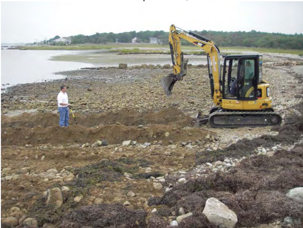
2. Trench excavation in cobble beach area – September 10, 2007.
