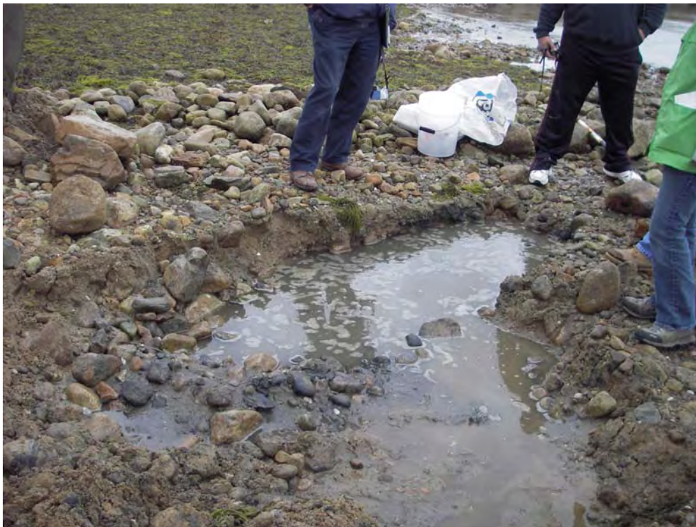
7. Cleanup activities in Area #1 – October 25, 2007.
