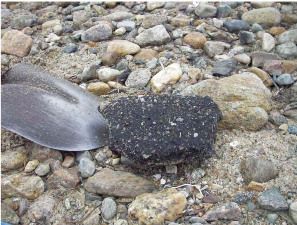
Reverse surface of roadway pavement noted above (note flat surface).
