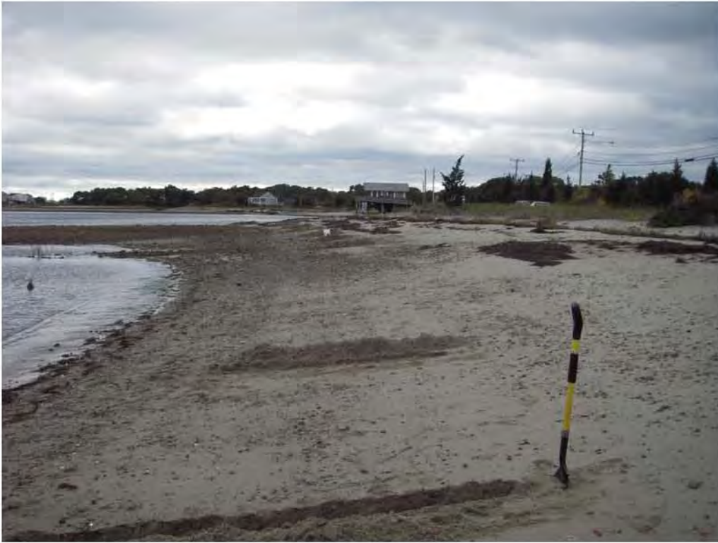
Trenches excavated along shoreline.
