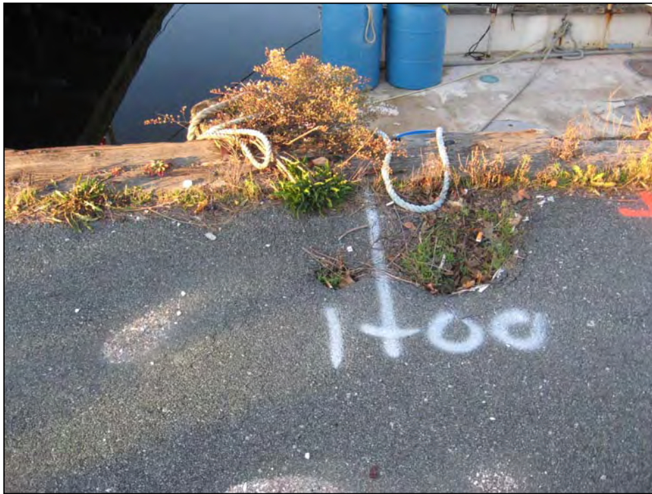
Photo No. 13: Area of subsidence behind the bulkhead wall. Note: Void observed in stone bulkhead in underwater inspection report.
