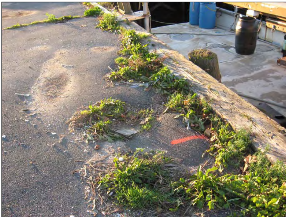
Photo No. 14: Areas of subsidence behind the bulkhead near Station 1+25.
