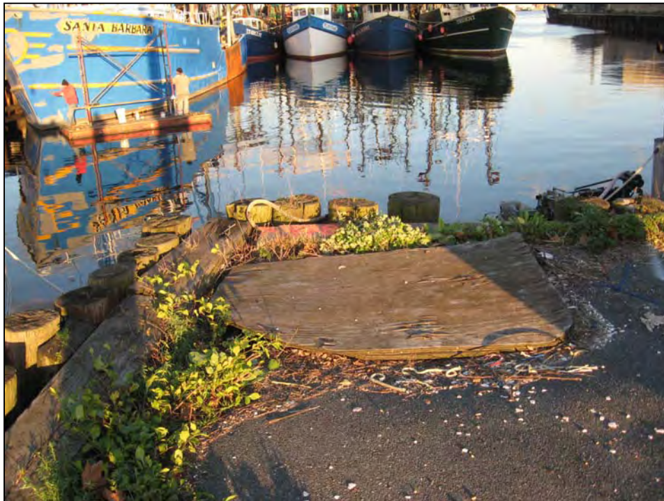
Photo No. 15: Plywood sheet covering 7' wide area of subsidence at Station 1+40.
