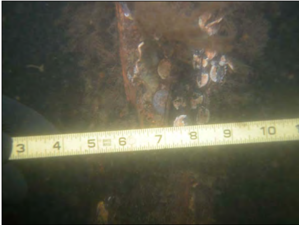
Photo No. 21: Typical underwater view of the timber pile section loss beneath the timber pier. (Photo by Childs Engineering Corp.)
