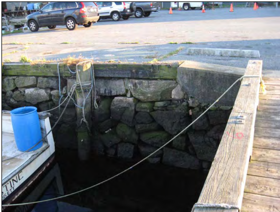
Photo No. 2: Typical stone bulkhead near Station 0+90.
