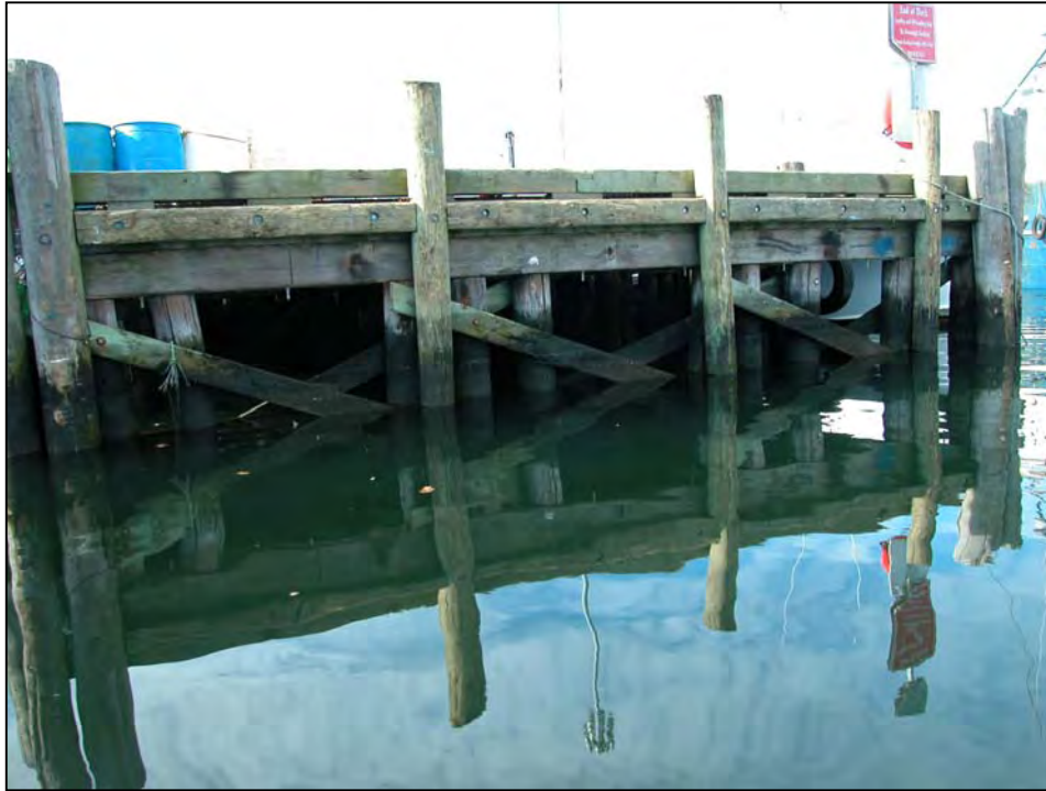
Photo No. 11: Overview of the end of the timber pier and timber fender system.
