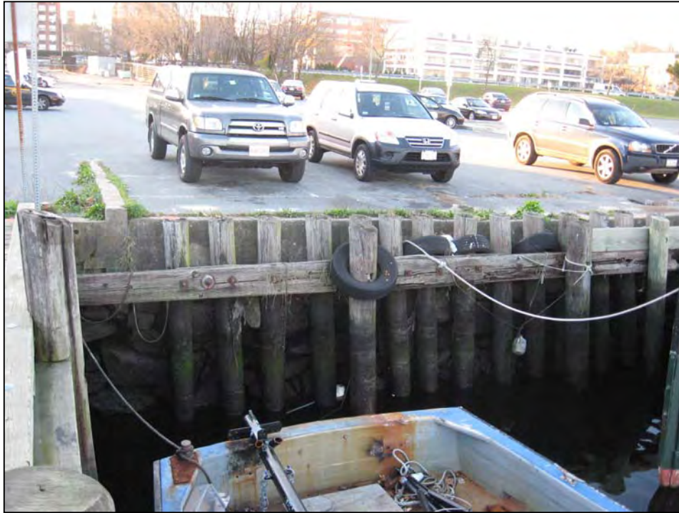
Photo No. 5: Timber fender system with docked vessel along the stone bulkhead from Station 1+70 to Station 2+10.
