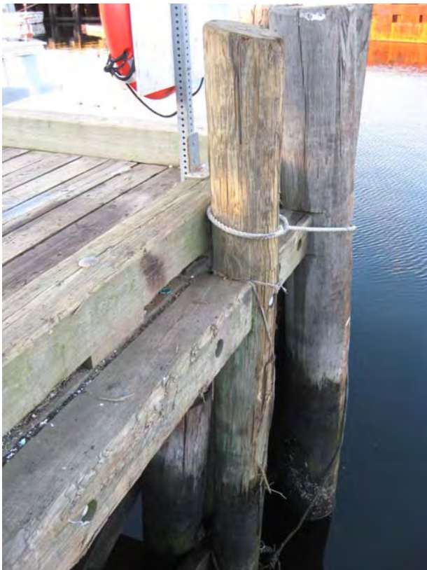
Photo No. 12: Typical wearing of the fender face at the end of the timber pier.
