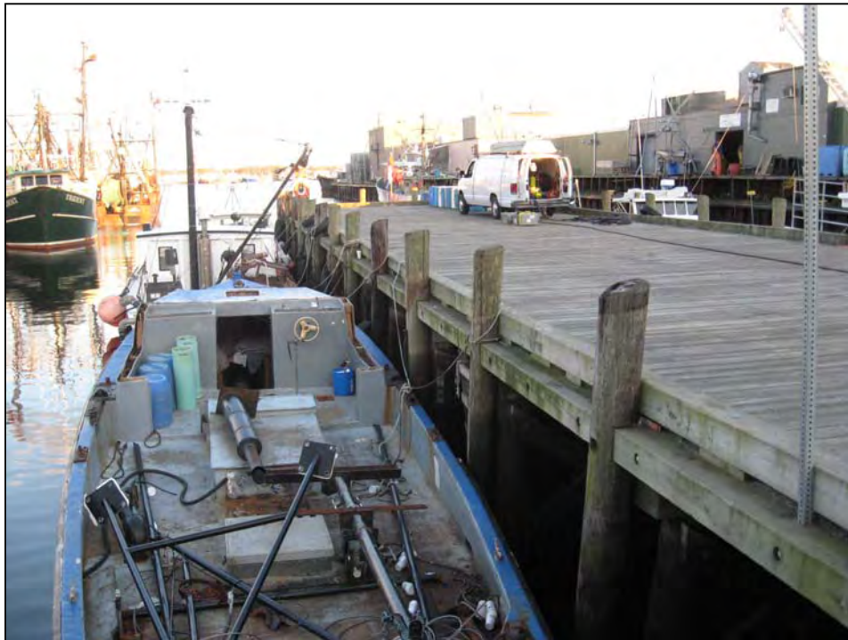
Photo No. 9: Overview of the fender system with docked vessel along the timber pier.
