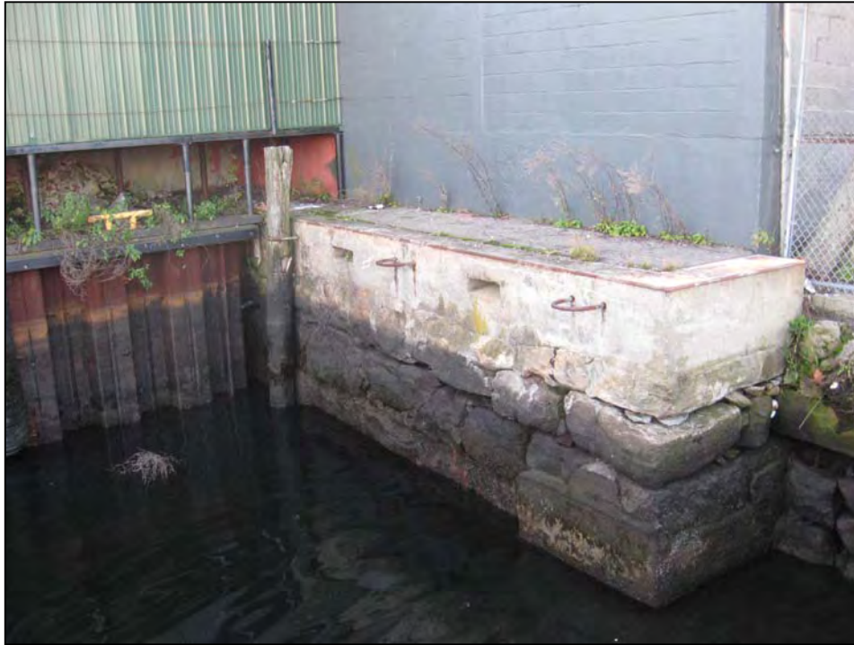
Photo No. 7: Stone bulkhead and concrete fill from Station 2+50 to Station 2+80.
