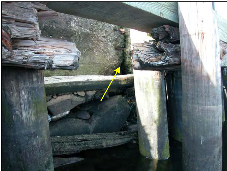
Photo No. 18: Displacement of the concrete wall with exposed reinforcement at Station 1+75.
