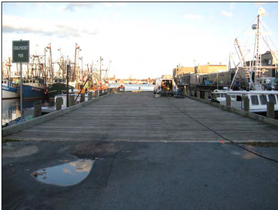
Photo No. 8: Overview of the 30' wide timber pile supported pier.
