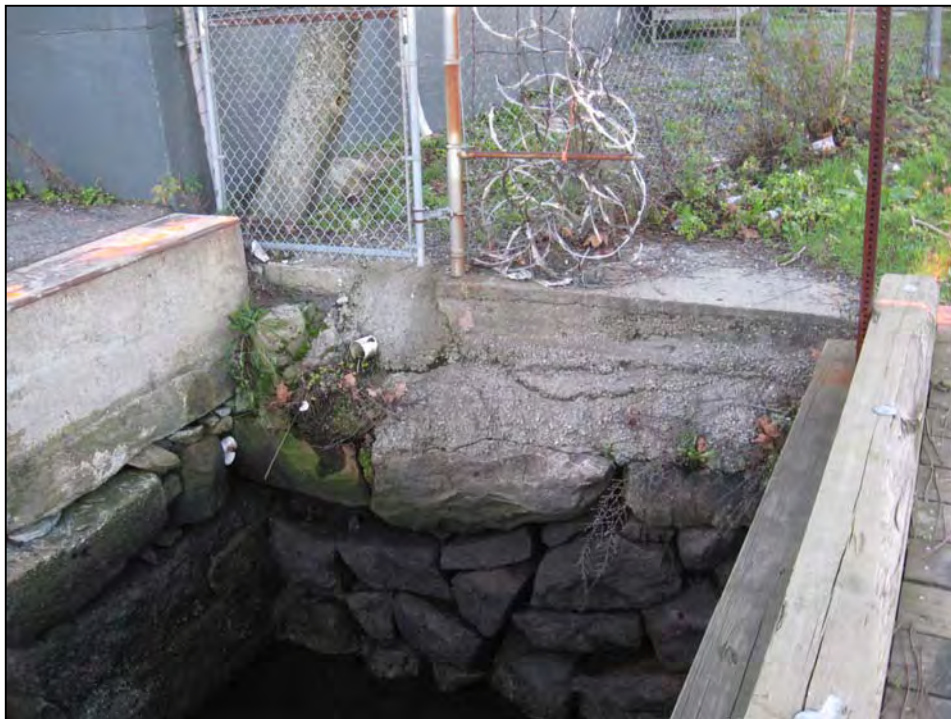
Photo No. 6: Stone bulkhead and concrete fill from Station 2+40 to Station 2+50.
