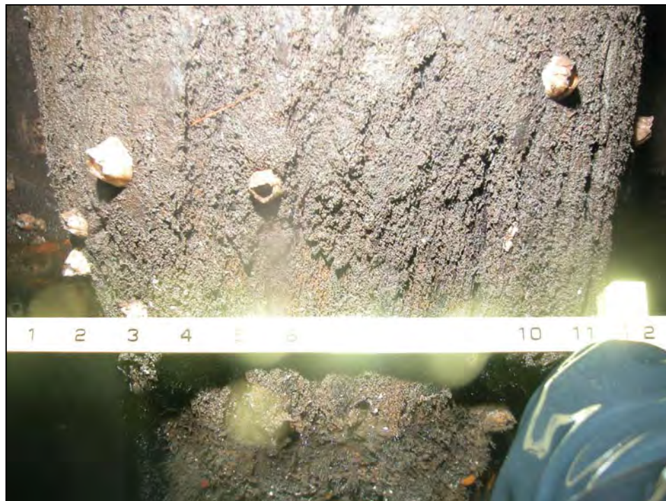
Photo No. 20: Typical underwater view of the timber pile section loss beneath the timber pier. (Photo by Childs Engineering Corp.)
