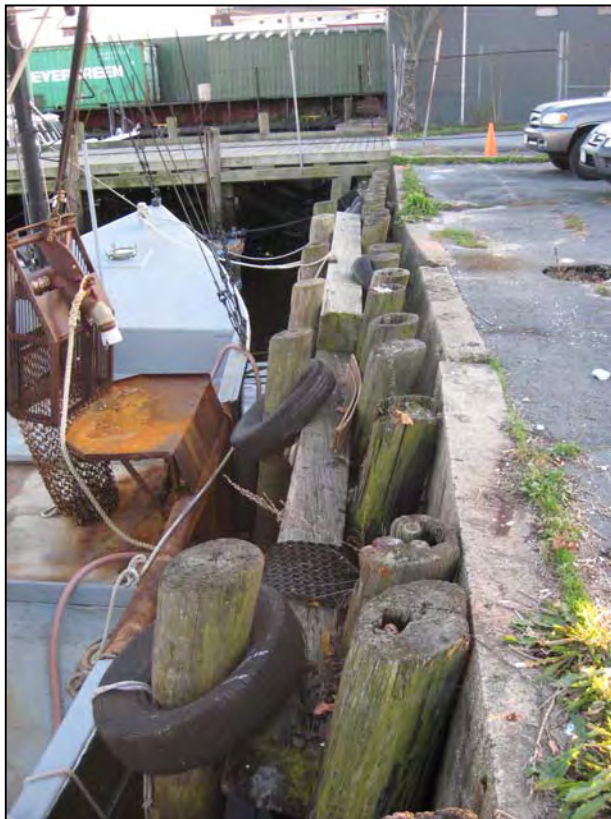
Photo No. 4: Timber fender system with docked vessel along the stone bulkhead from Station 1+33 to Station 2+10.
