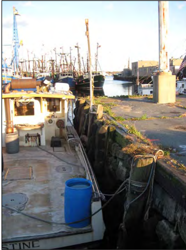
Photo No. 3: Timber fender piles with docked vessel along the stone bulkhead from Station 0+86 to Station 1+33.
