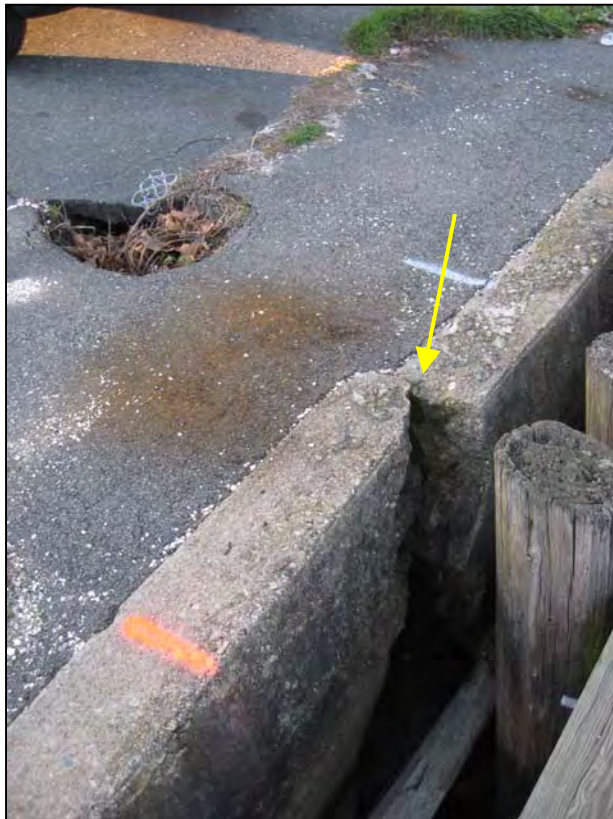
Photo No. 17: Area of subsidence (34" diameter) at Station 1+76. Note the displacement of the concrete wall.
