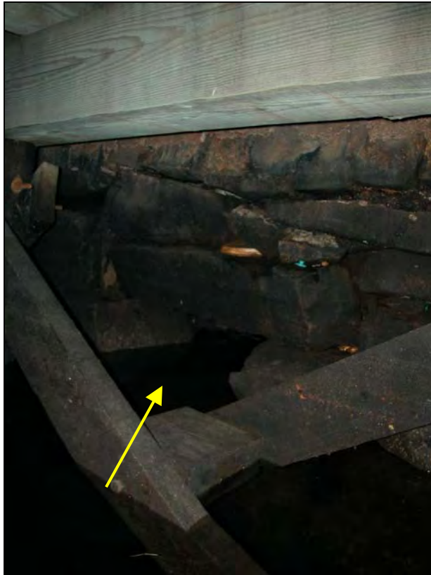
Photo No. 19: Void observed in the stone bulkhead at Station 2+20 beneath the timber pier
