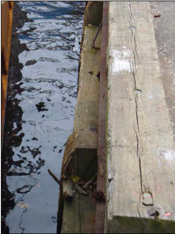
Photo No. 5: Typical worn fender pile with missing UHMW rub rail.
