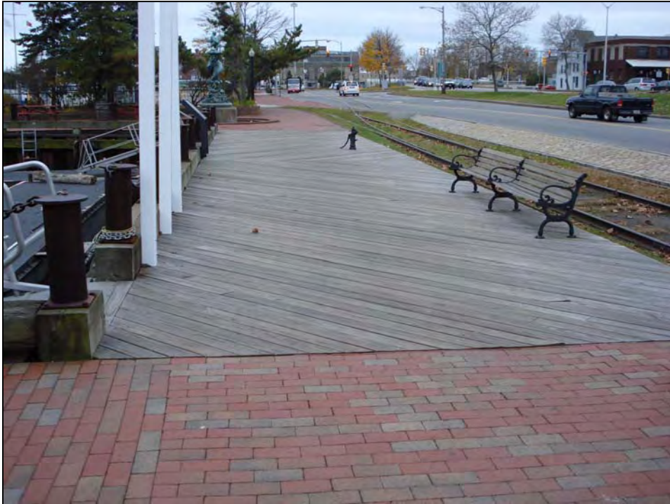
Photo No. 15: Overview of the timber deck from Station 10+44 to Station 11+21.
