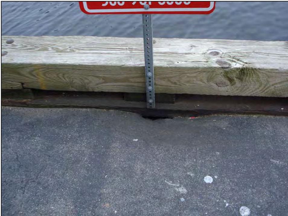
Photo No. 18: Subsidence behind the steel sheetpile bulkhead at Station 9+34.
