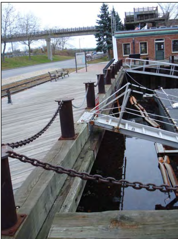
Photo No. 16: Overview of the timber curb with steel bollards along the timber deck.
