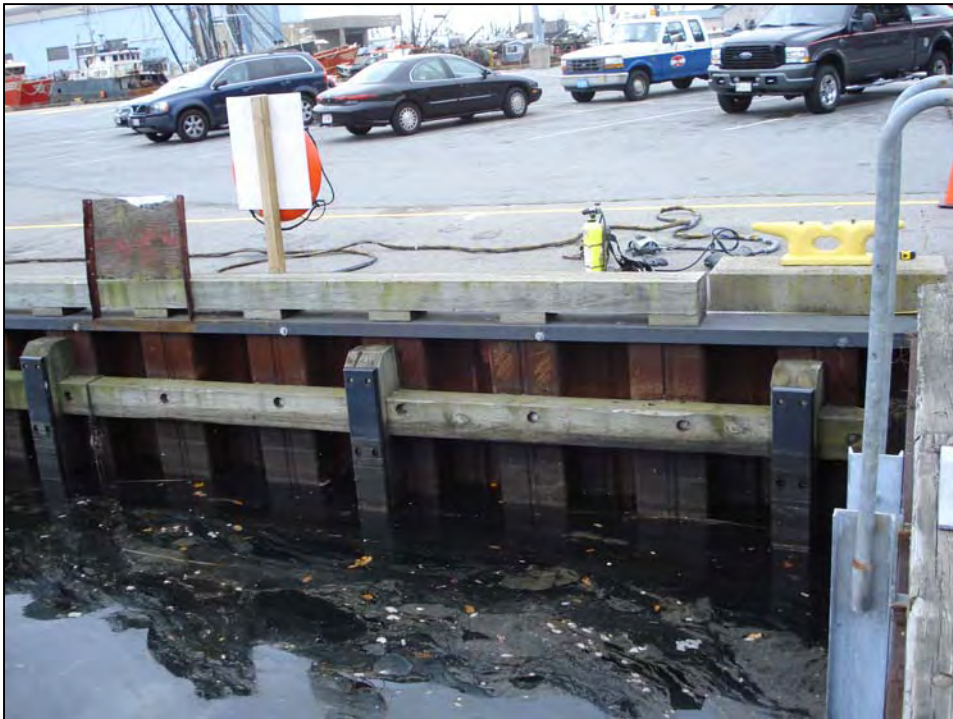
Photo No. 3: Typical overview of the timber fender system with UHMW rubber rails.
