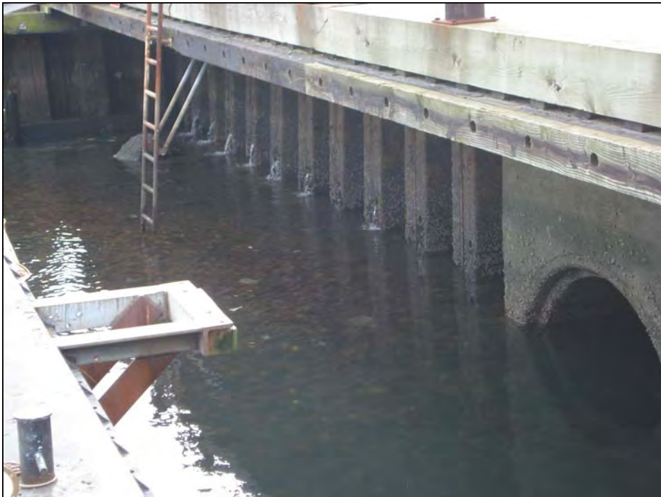
Photo No. 14: Overview of the steel sheetpile bulkhead beneath the timber deck from Station 10+44 to Station 11+21.
