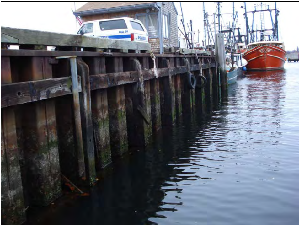
Photo No. 12: Overview of the older fender system from Station 8+84 to Station 10+44.
