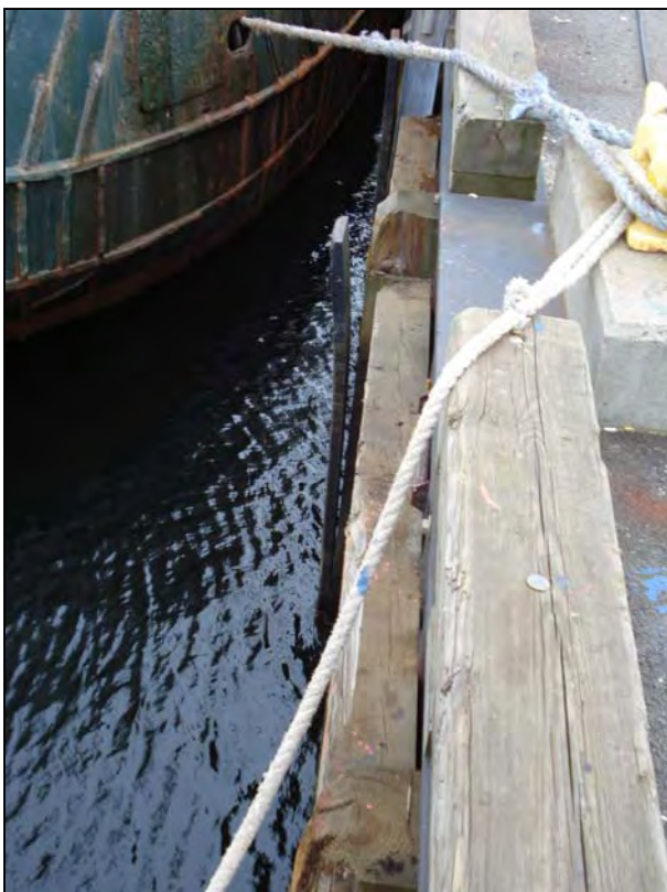
Photo No. 6: Typical loose UHMW rub rail.
