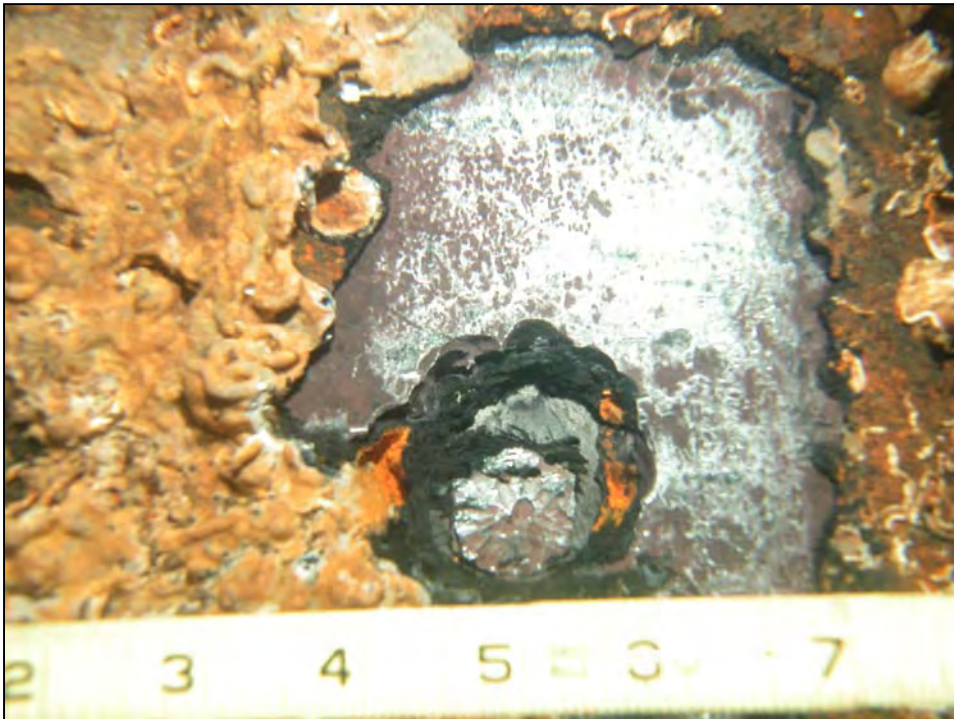
Photo No. 19: Observed steel sheetpile condition underwater (Photo by Childs Engineering Corp.)
