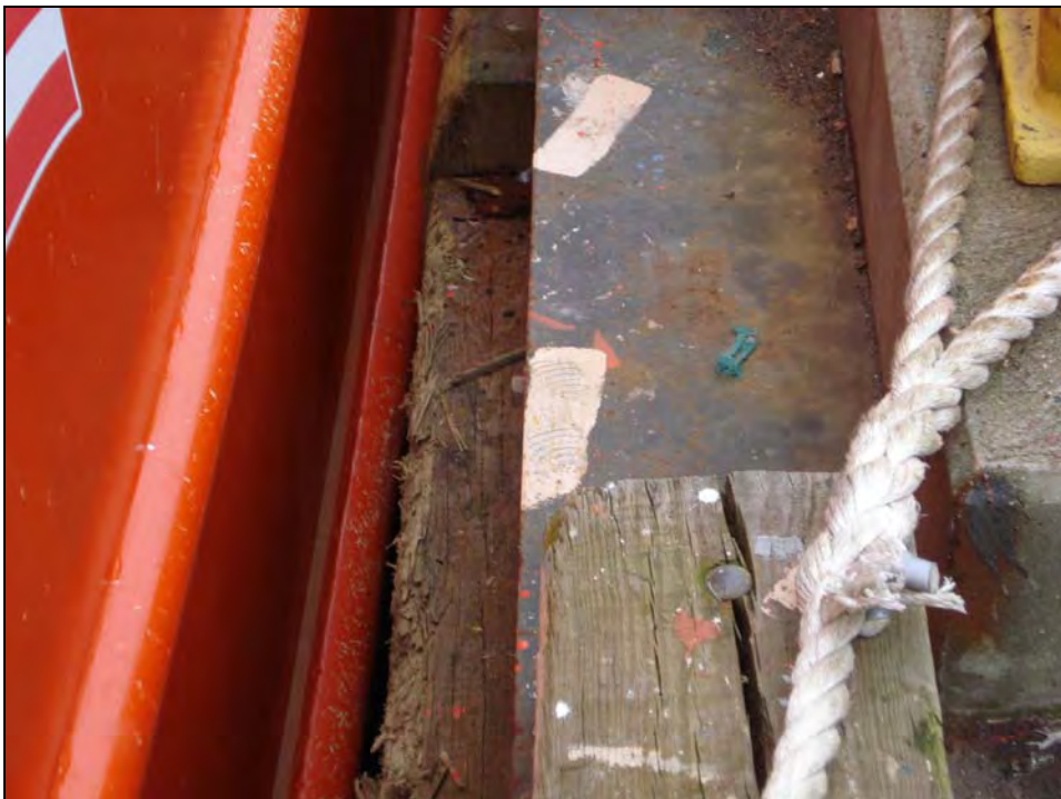
Photo No. 8: Worn fender pile in contact with a docked vessel.
