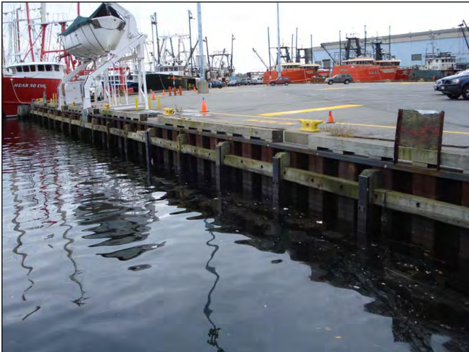
Photo No. 2: Steel Sheetpile bulkhead from approximately Station 0+20 to Station 1+73.
