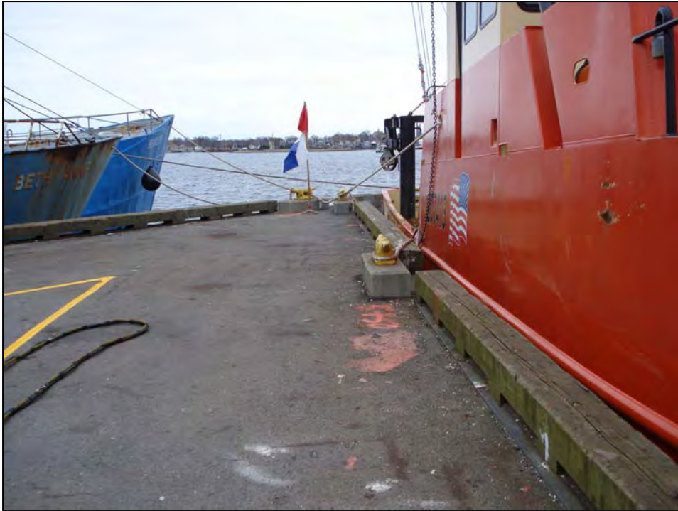
Photo No. 9: Overview of the eastern corner of the wharf.
