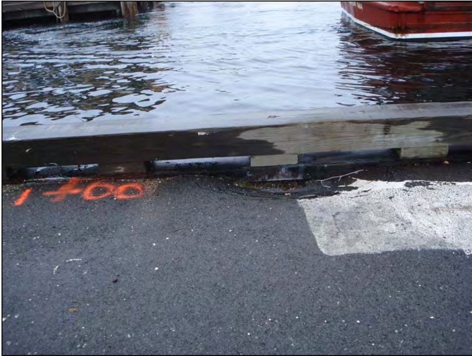
Photo No. 17: Subsidence behind the steel sheetpile bulkhead at Station 1+06.
