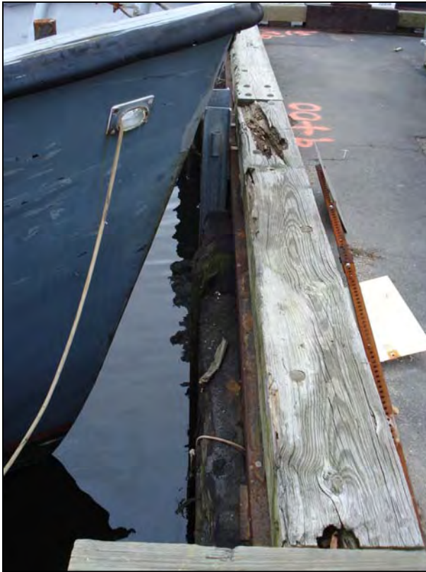
Photo No. 13: Older fender system with rotted timber curb and damaged chocks.
