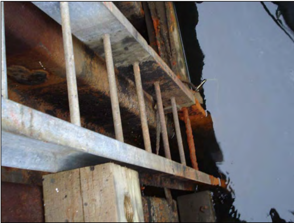
Photo No. 11: Typical access ladder with corroded rungs.
