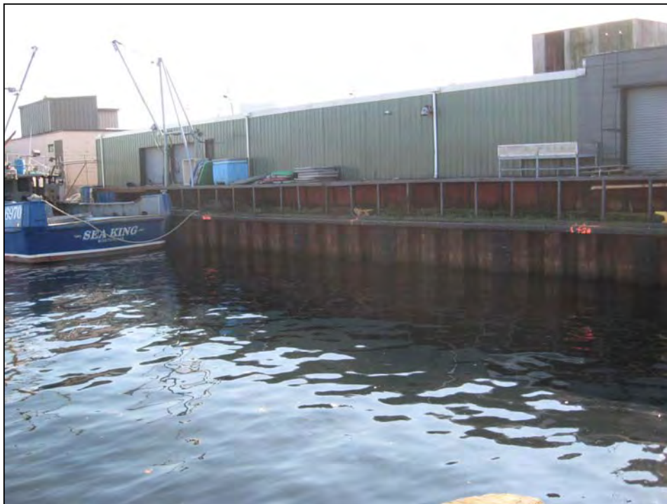
Photo No. 2: Overview of the sheetpile bulkhead and rubber tire fender system from Station 1+50 to Station 2+00.
