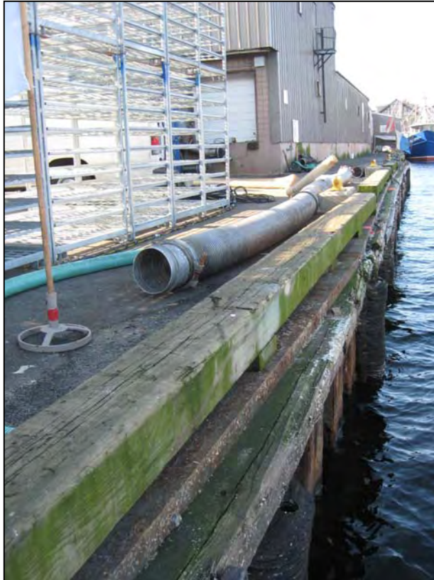
Photo No. 7: Timber wale with missing UHMW rub rail. Note the damage to the wale.
