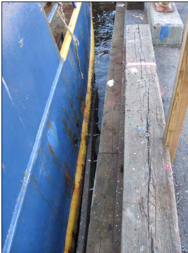
Photo No. 14: Typical loose UHMW rubber rail near Station 7+75.
