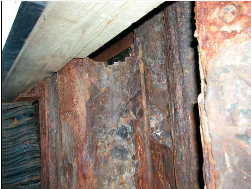
Photo No. 10: Hole in steel sheet pile bulkhead at Station 5+93.
