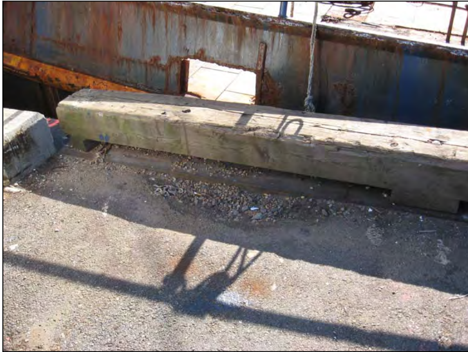
Photo No. 13: Subsidence behind the sheetpile bulkhead at Station 7+57.
