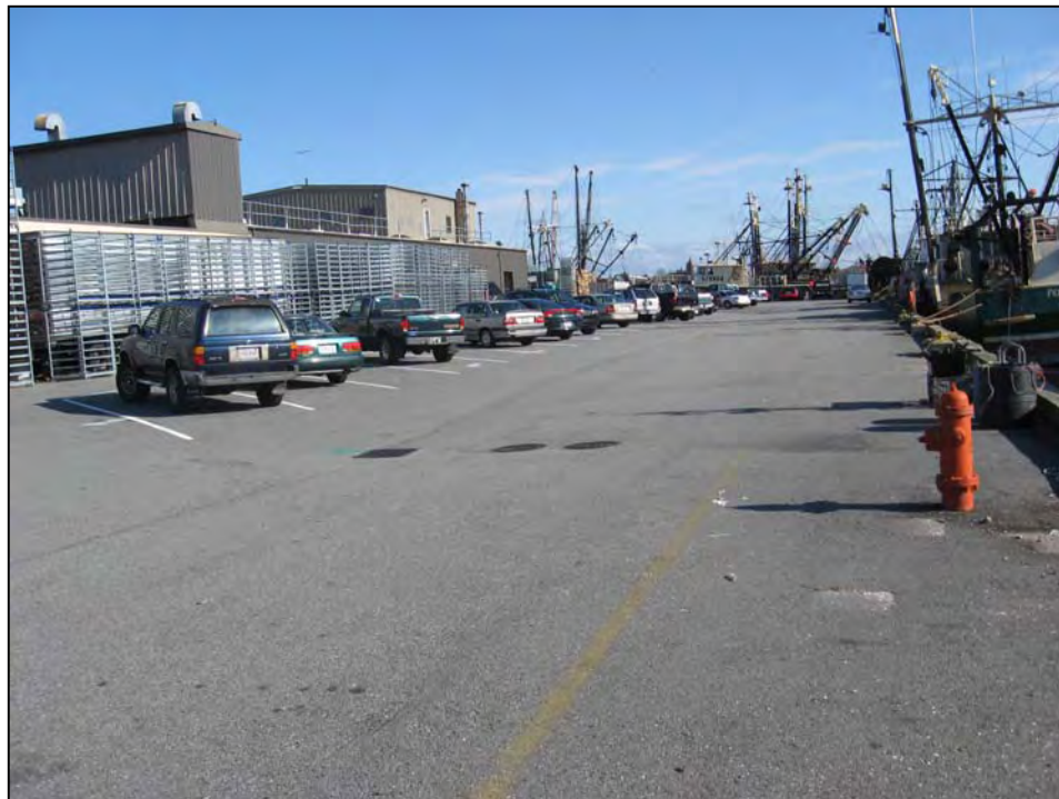
Photo No. 20: Overview of the bituminous deck and parking area.
