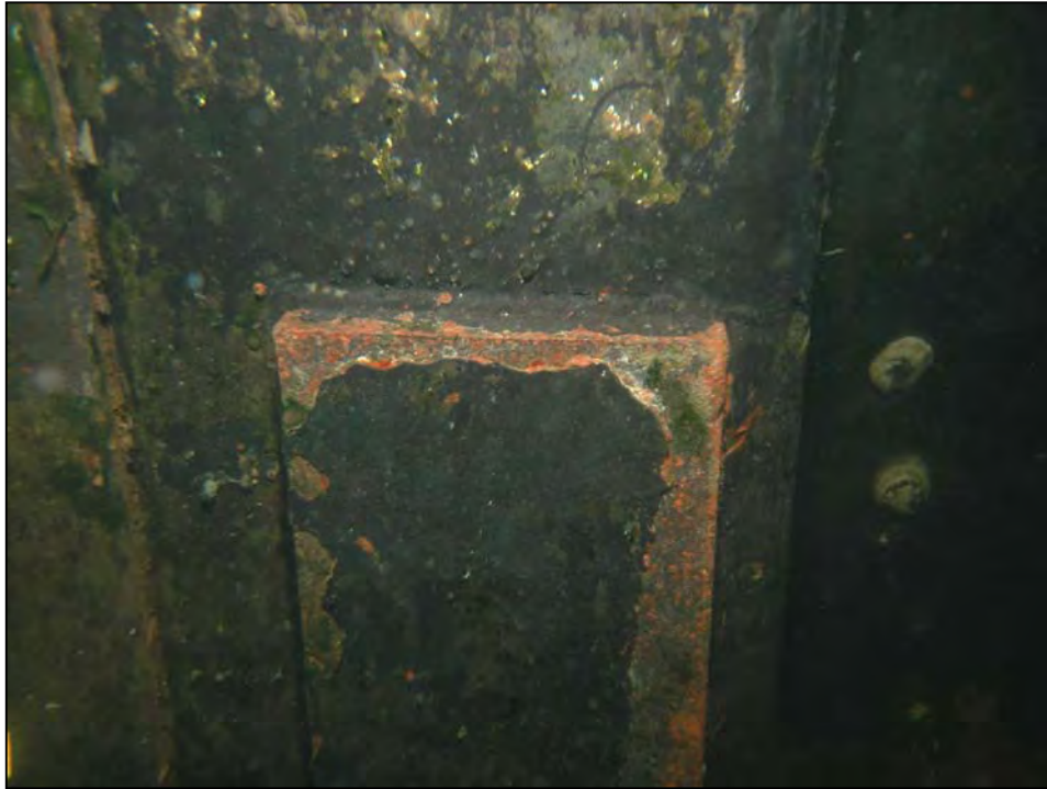
Photo No. 21: Typical steel face plate mounted to steel sheetpile. (Photo by Childs Engineering Corp.)
