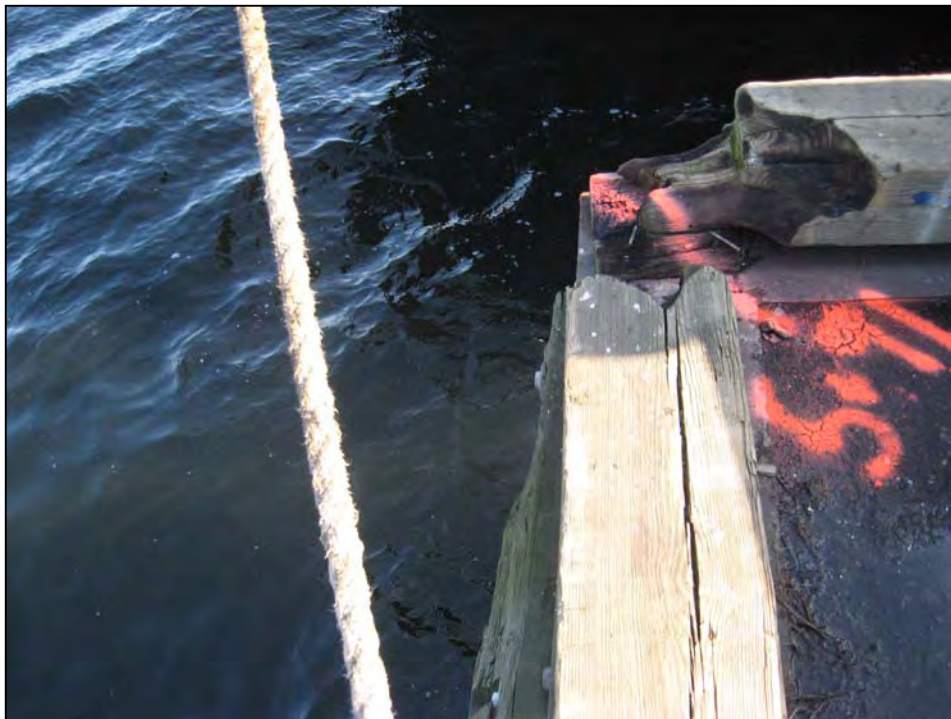
Photo No. 8: Fire damage on the timber curb at the corner of the bulkhead at Station 5+91.
