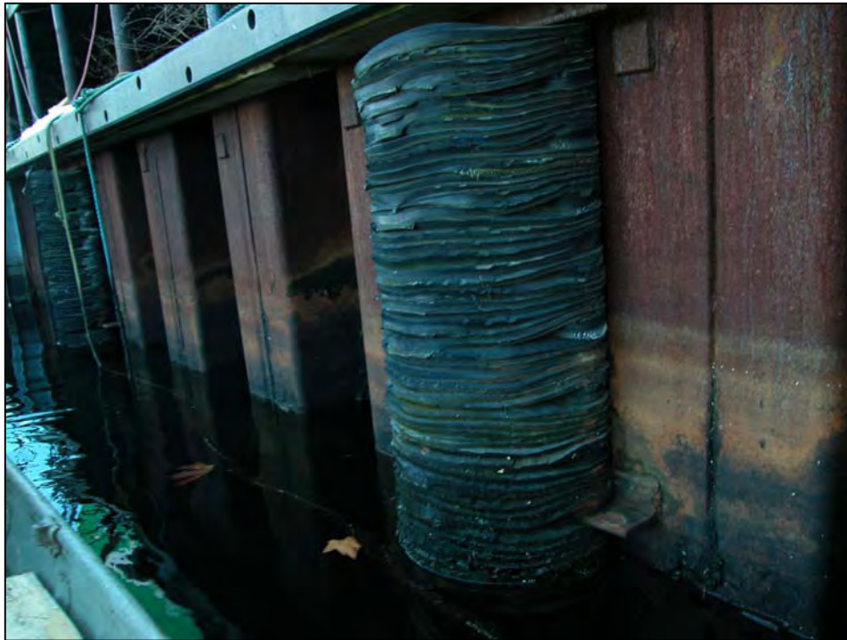
Photo No. 3: Typical rubber tire fender with steel brackets along the steel sheetpile bulkhead.
