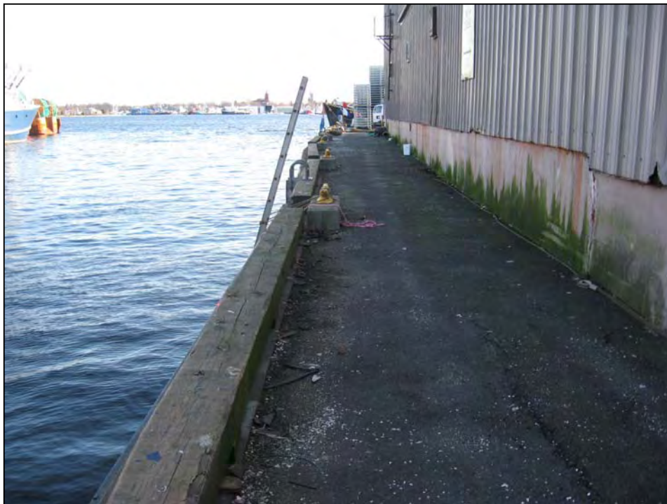
Photo No. 6: Bituminous deck with timber curb looking east.
