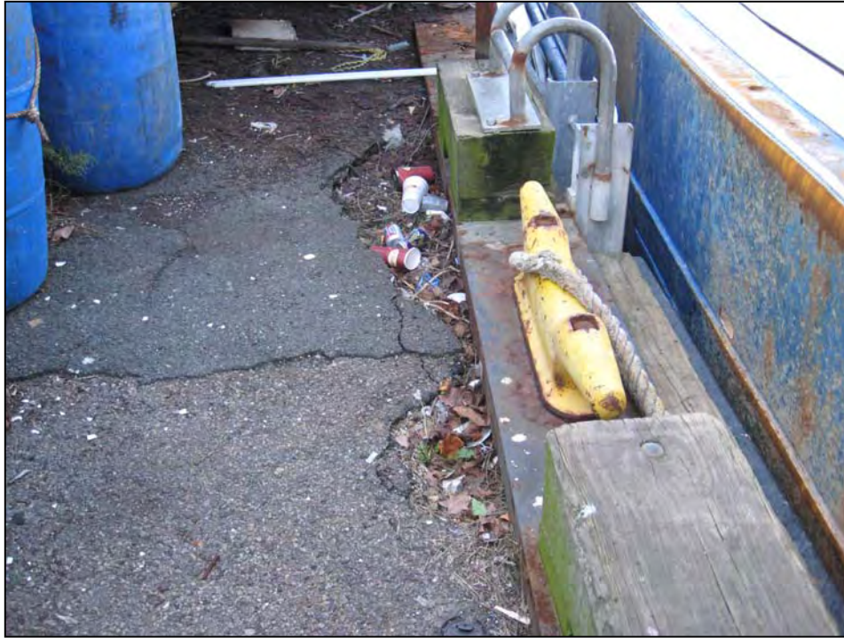
Photo No. 5: Subsidence behind the sheetpile bulkhead at Station 2+35 to Station 2+40.
