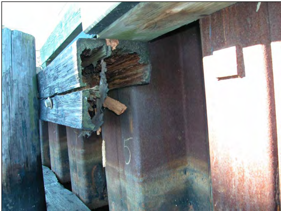
Photo No. 16: End of rotted top wale of the old timber fender system.
