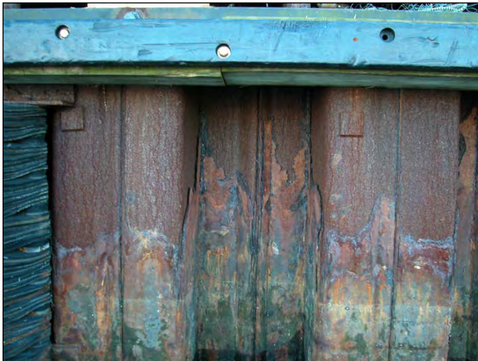
Photo No. 4: Typical condition of the sheetpile bulkhead.
