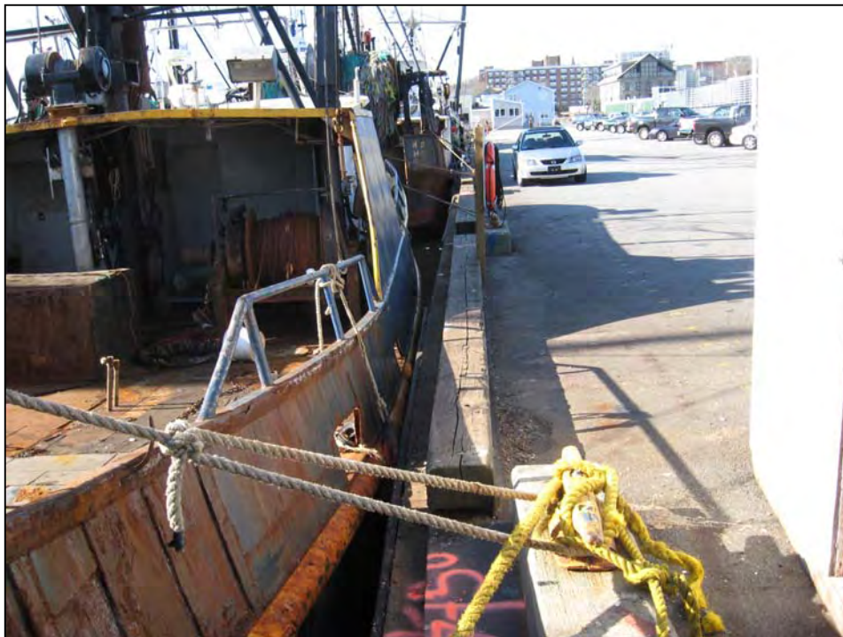
Photo No. 12: Overview of the timber curb and bituminous deck from Station 7+50 looking west.
