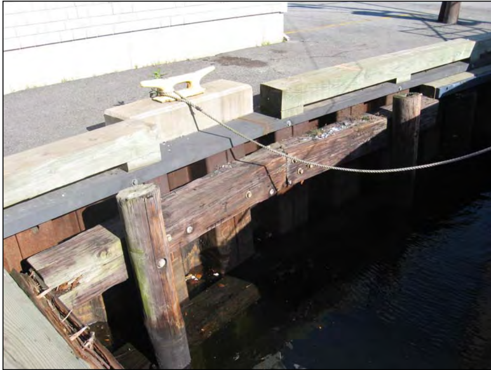
Photo No. 15: Old timber fender system starting at Station 11+70.
