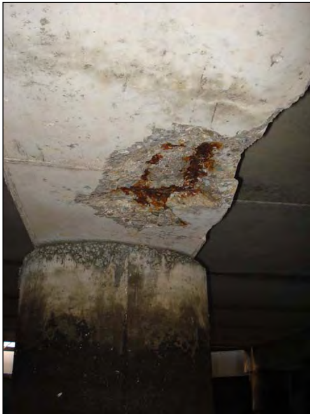
Photo No. 22: Typical spalling of the underside of the pile cap beneath the original pier structure.
