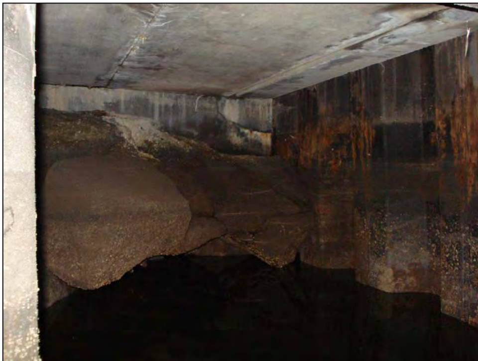
Photo No. 30: Overview of the void at the corner of the granite block wall and the steel sheetpile bulkhead under the timber boardwalk.
