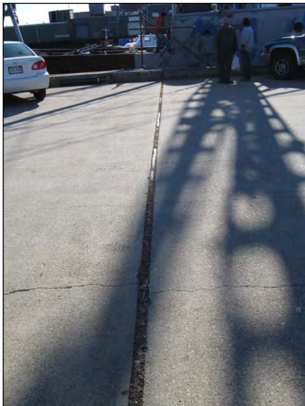
Photo No. 6: Typical expansion joint in the deck of the original structure. Note missing joint sealer.
