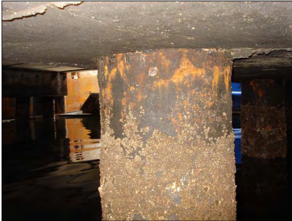
Photo No. 25: Typical top of pile at the intersection of the concrete pile cap beneath the pier extension.
