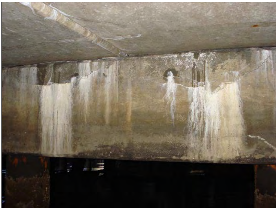
Photo No. 20: Typical spalling of the pile cap beneath the pier extension. Note presence of efflorescence.
