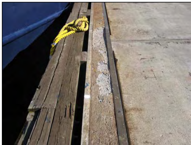
Photo No. 12: Spalling of concrete on top and face of curb.
