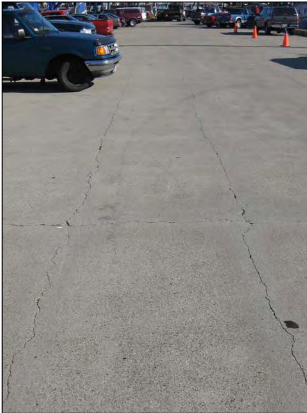
Photo No. 3: Typical longitudinal and transverse cracking observed along the deck of the original structure.
