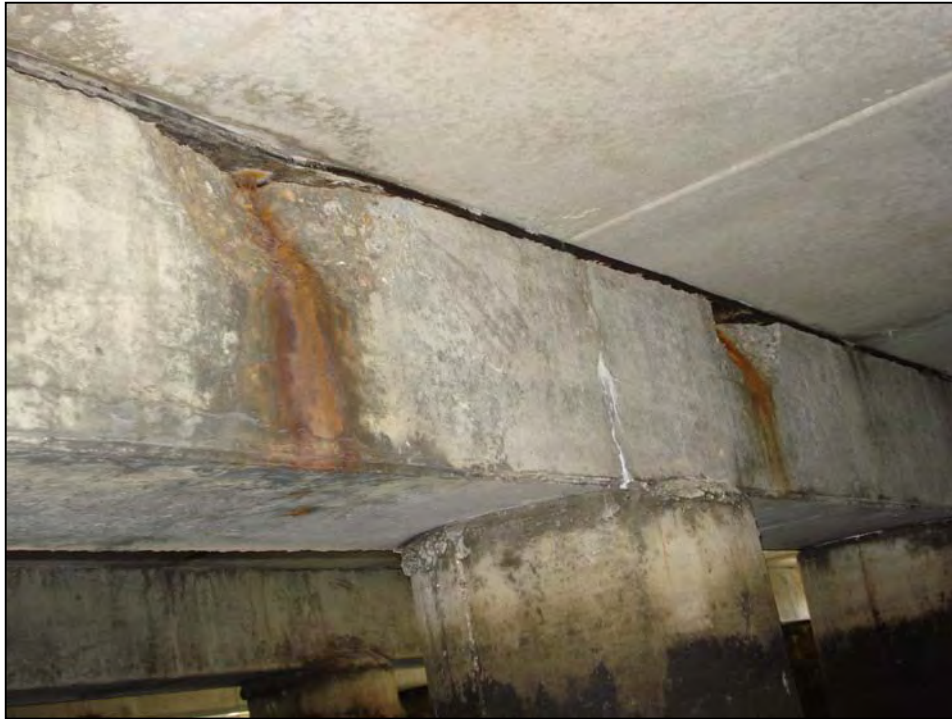
Photo No. 23: Spalled areas on the concrete pile cap with rust staining from exposed steel reinforcement.
