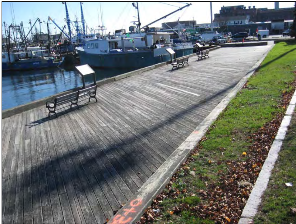
Photo No. 1: Timber wharf from Station 0+00 to Station 1+54.
