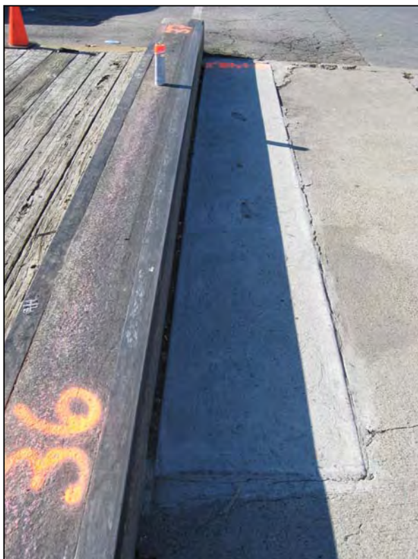
Photo No. 18: Patch in the southwest corner of the concrete deck.
