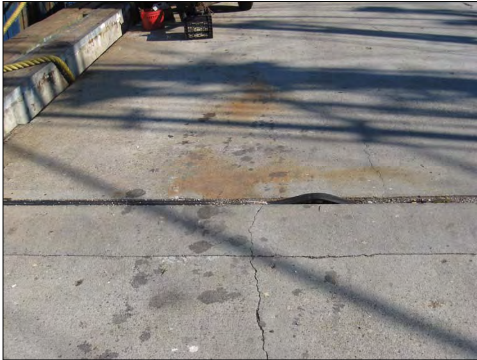
Photo No. 7: Loose joint filler at intersection of original structure and pier extension.
