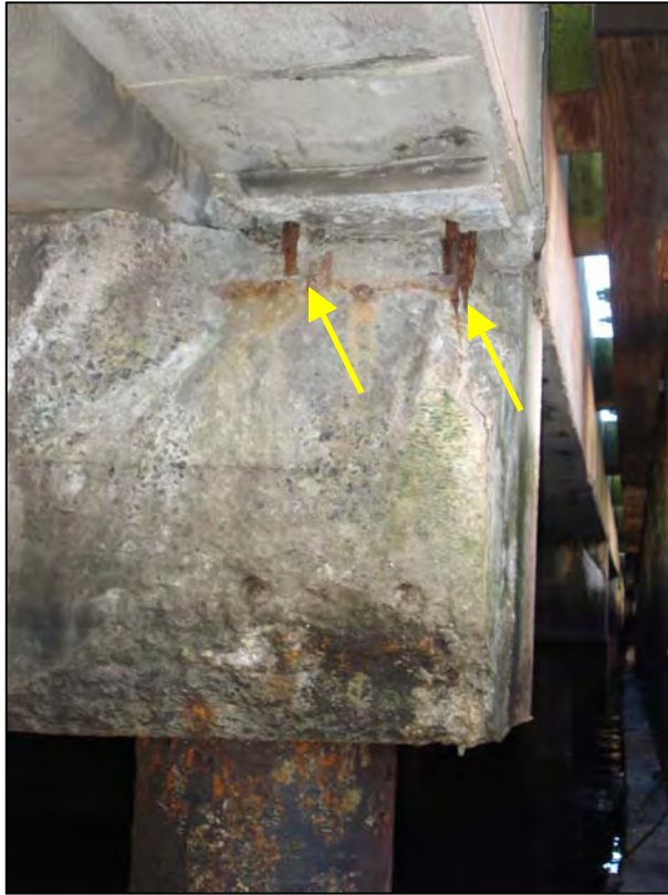
Photo No. 21: Significant spalling of the concrete pile cap along the waterside edge beneath the original pier structure. Note exposed reinforcement.
