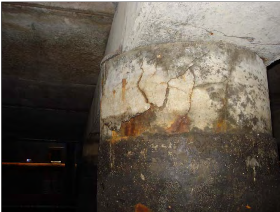
Photo No. 24: Cracking at the top of the concrete pile beneath the original pier structure.
