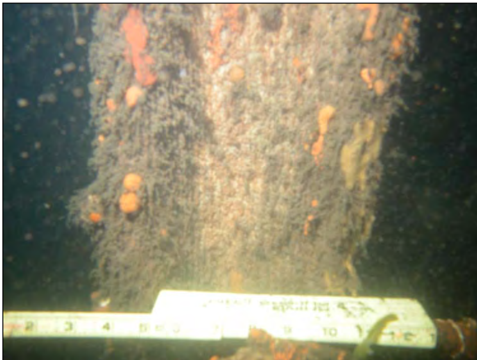
Photo No. 34: Underwater photo of marine growth on the pile. (Photo by Childs Engineering Corp.)
