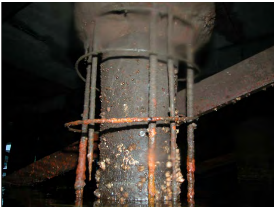
Photo No. 26: Missing concrete jacket with exposed steel reinforcement cage and timber pile. (Photo by Childs Engineering Corp.)
