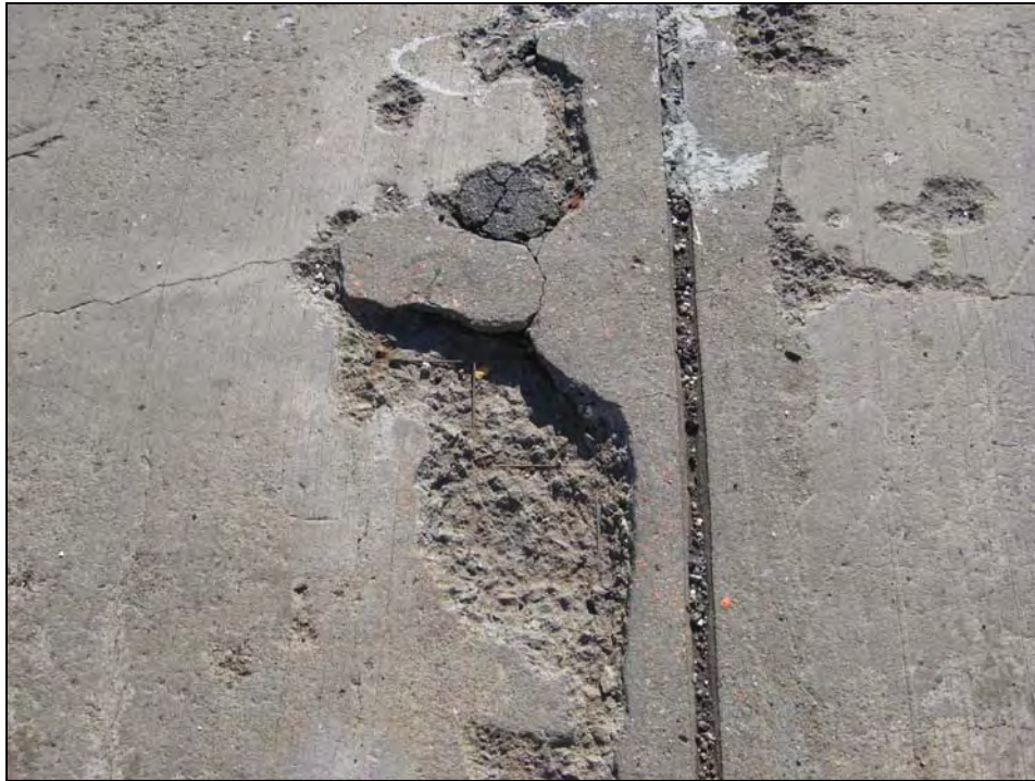
Photo No. 11: Spalling of the concrete deck with exposed reinforcement observed in several locations.
