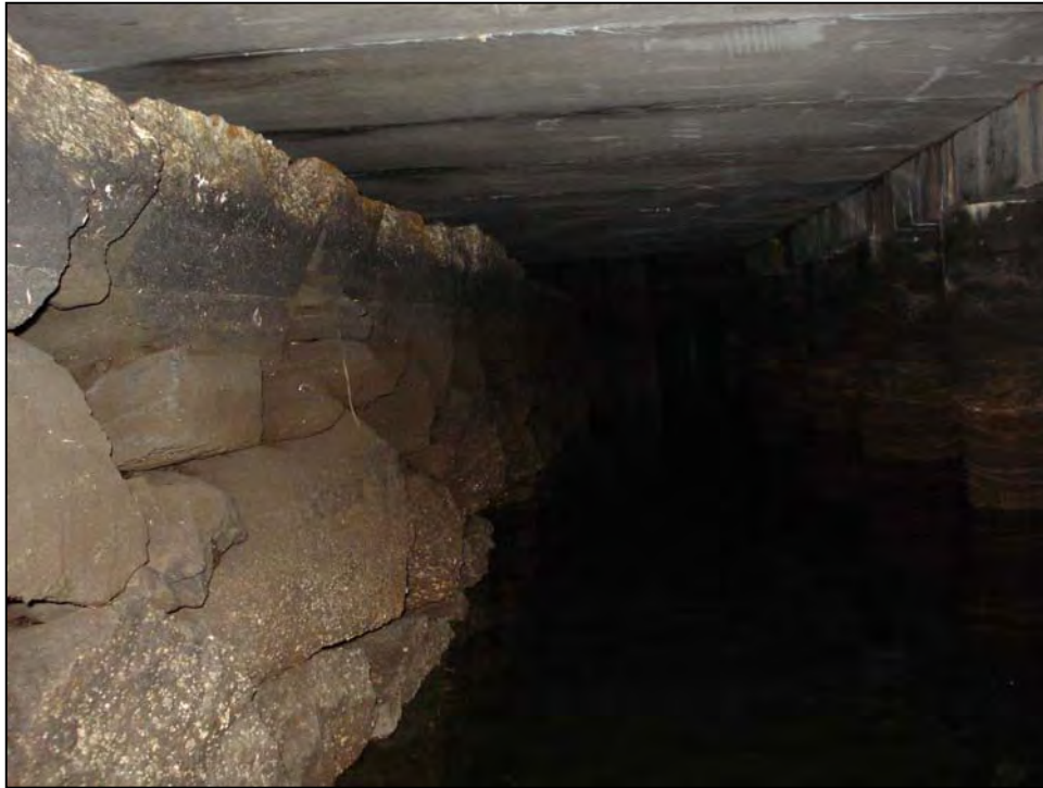
Photo No. 29: Overview of the granite block wall along the shoreline beneath the original structure looking north.
