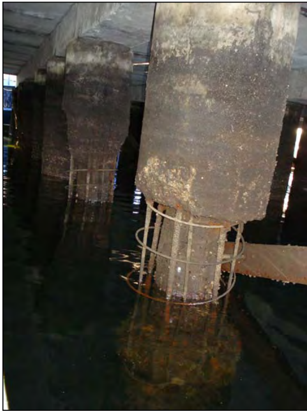
Photo No. 27: Missing concrete jacket with exposed steel reinforcement cage and timber pile.
