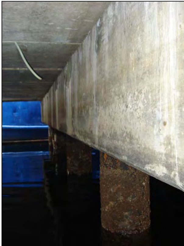
Photo No. 19: Typical overview of the deck slabs, concrete pile caps, and piles below the pier extension.
