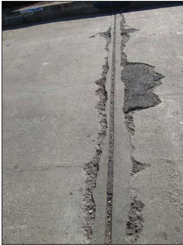
Photo No. 9: Typical expansion joint in the deck of the pier extension. Note spalling of concrete and asphalt patch.
