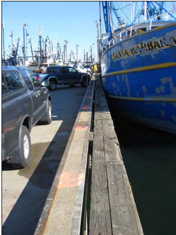
Photo No. 17: Overview of the curb and fender system on the south face of the pier.
