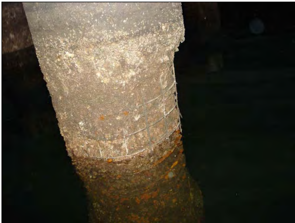
Photo No. 28: Missing concrete jacket with exposed steel reinforcement cage in the tidal zone.
