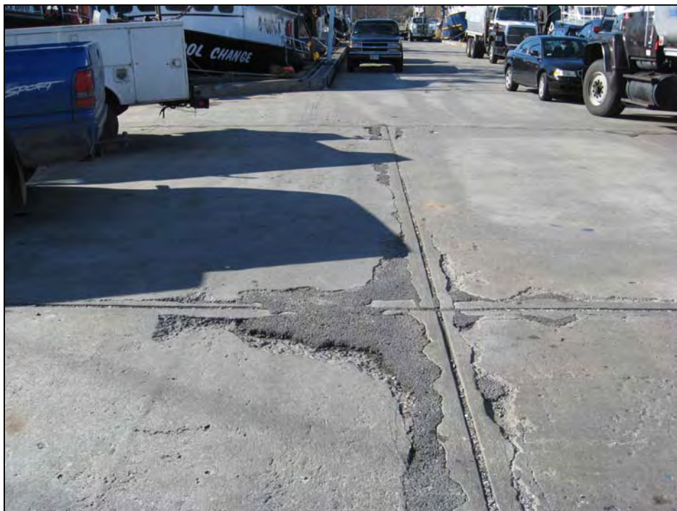
Photo No. 10: Four way intersection of expansion joints at the head of the pier extension.
