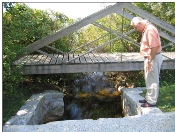
Figure 76. This water level control structure at Cockeast Pond, Westport was modified to enhance herring passage.
