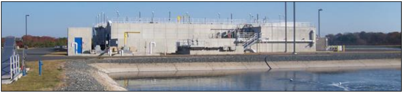
Figure 27. Town of Falmouth wastewater facility.
