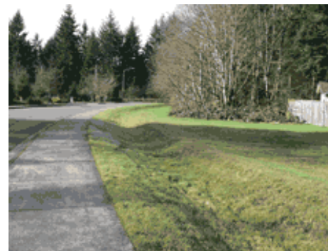
Stormwater can be directed to swales and biofilters along the edge of a road, where some of the water can soak into the ground.
