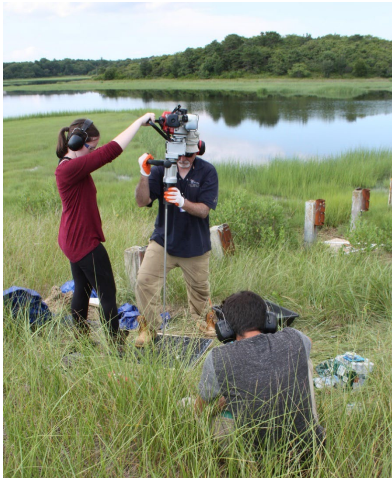
Installation of an elevation benchmark
