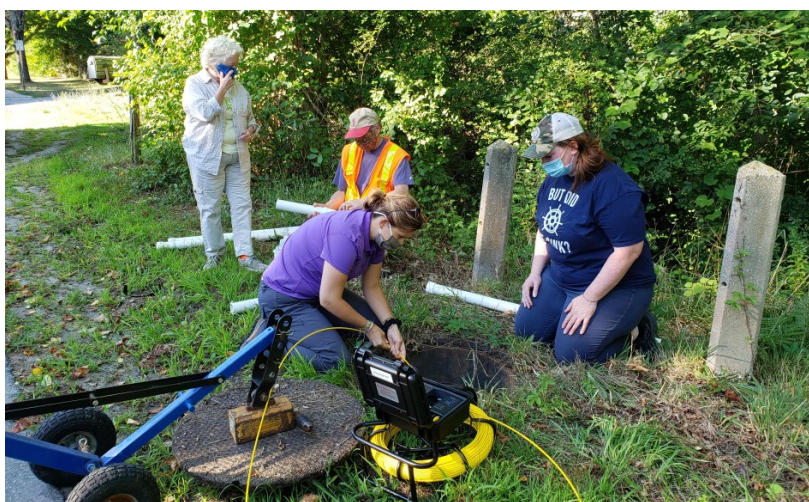
Fig. 6 NEP and MMA staff trained Marion DPW on the use of the newly outfitted IDDE trailers.
