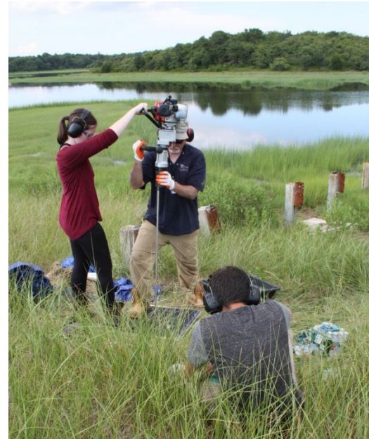
Fig. 15 Between 2019 and 2021, the NEP oversaw the installation NGS rod type elevation benchmarks at 12 long-term salt marsh study sites in Buzzards Bay.
