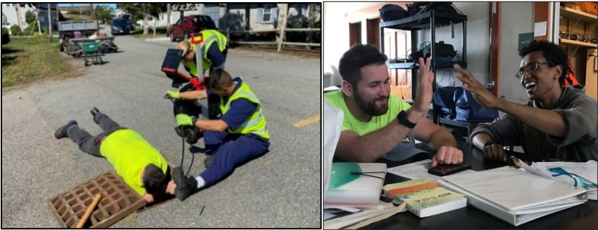
Co-op students deploying the camera inspection system (left), and finishing an assignment (right).
