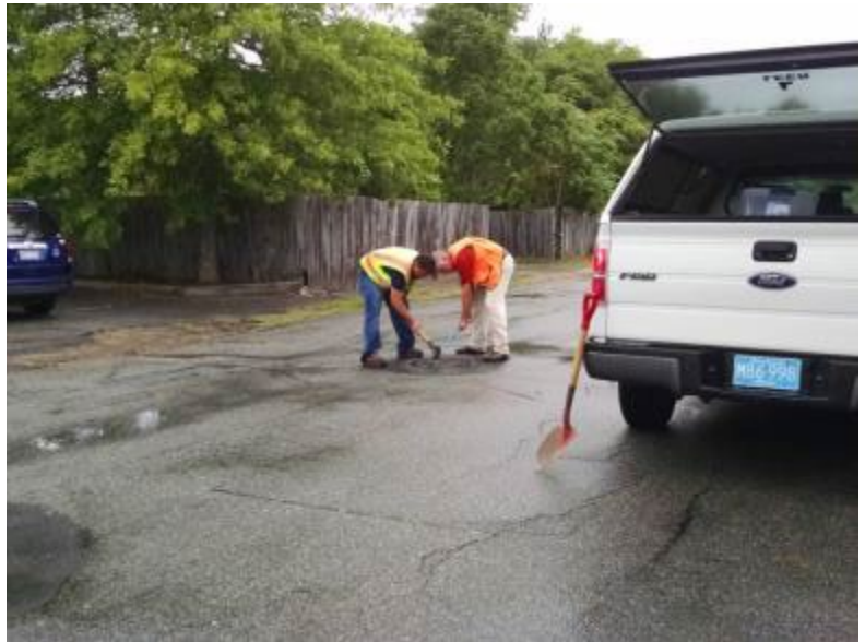
Fig. 8. Manhole covers must be removed to confirm network connections and for sampling.
