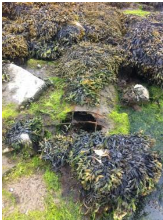
Fig. 7. Many discharges are intertidal or subtidal. Even when they can be sampled at low tide, the sample may be mostly salt water that intruded into the pipe.
