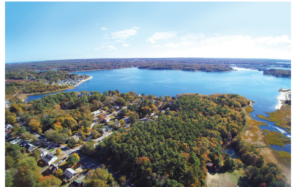
Buttermilk Bay is one of the estuaries that would benefit most from a regional sewer approach.
