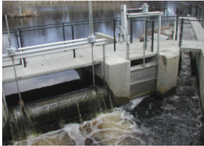
Dam at Route 6 Crossing
