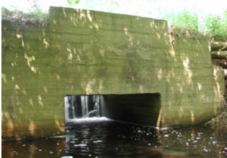
Rochester Fish Hatchery Dam
