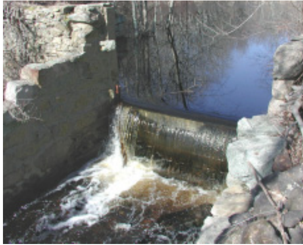
Dam at Rounseville Road Crossing
