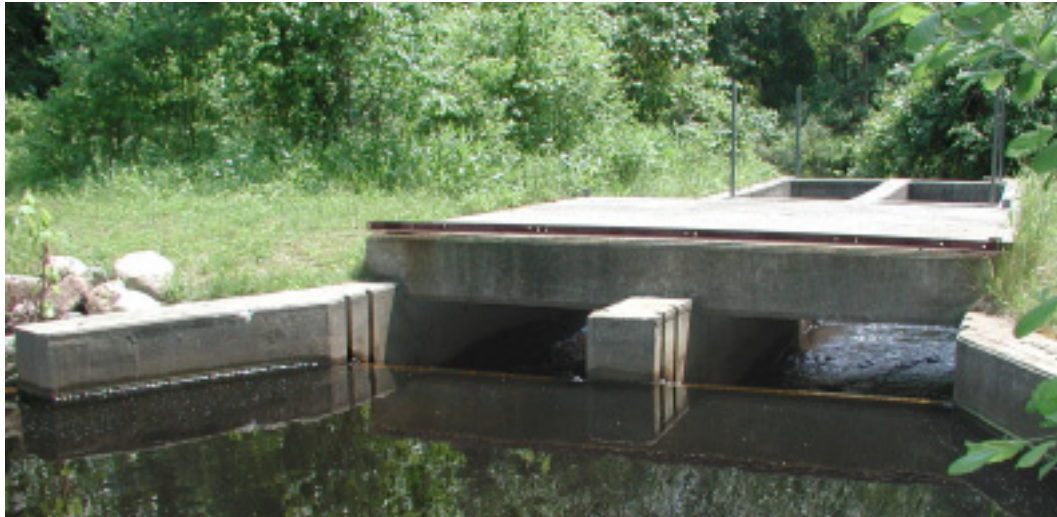
Snipatuit Pond Dam and Ladder
