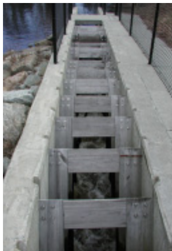
Ladder at Route 6 Crossing
