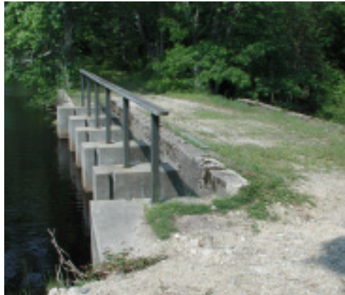
Hathaway Pond Dam
