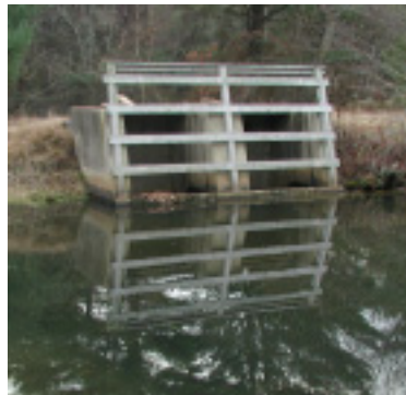
Bog Sluice at base of impoundment Upstream of Tihonet Pond
