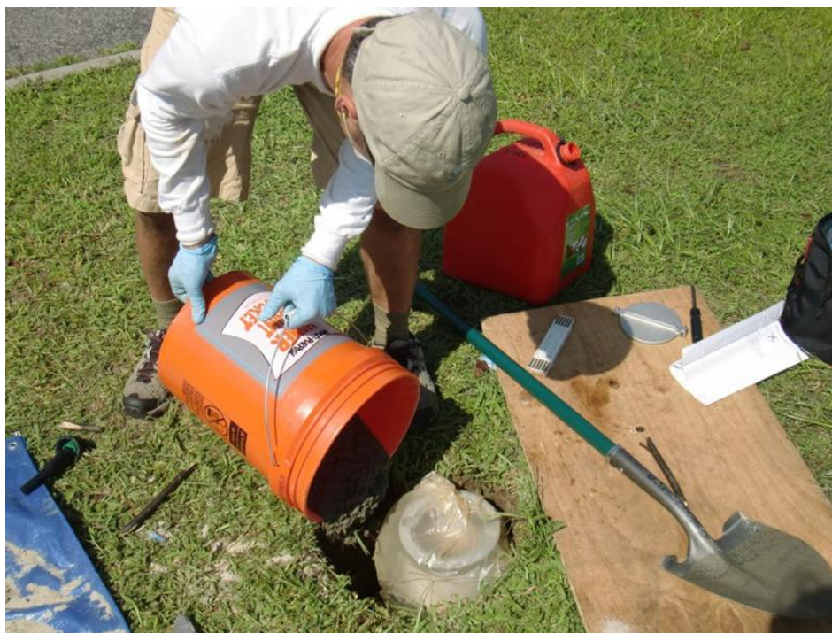
Fig. 33. Use a plastic bag to protect the access cover from the poured concrete.
