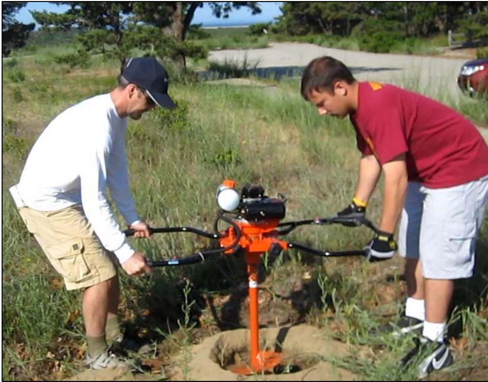
Fig. 25. Using a power auger (pictured) or spade, dig a hole 42" deep.
