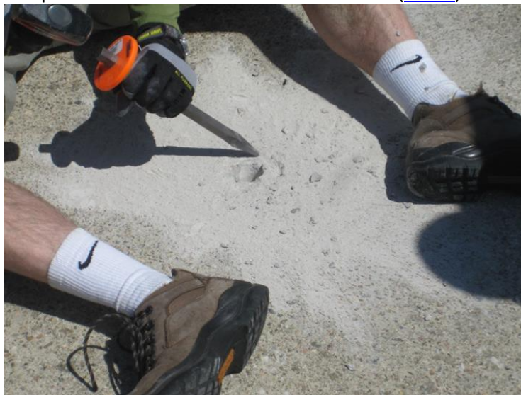
Fig. 24. Figure 7. Using a hammer and a chisel, chip away at the substrate to recess the disk ( video 1 , video2 ).
