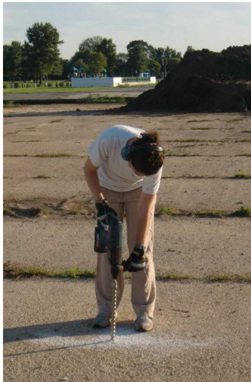
Fig. 23. Figure 6. Drill a hole using a cordless hammer drill. A sharp drill bit and extra batteries are essential ( video ).
