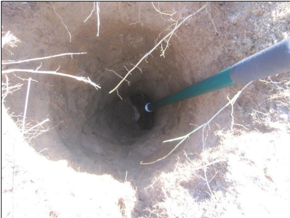
Fig. 25. Using a power auger (pictured) or spade, dig a hole 42" deep.
