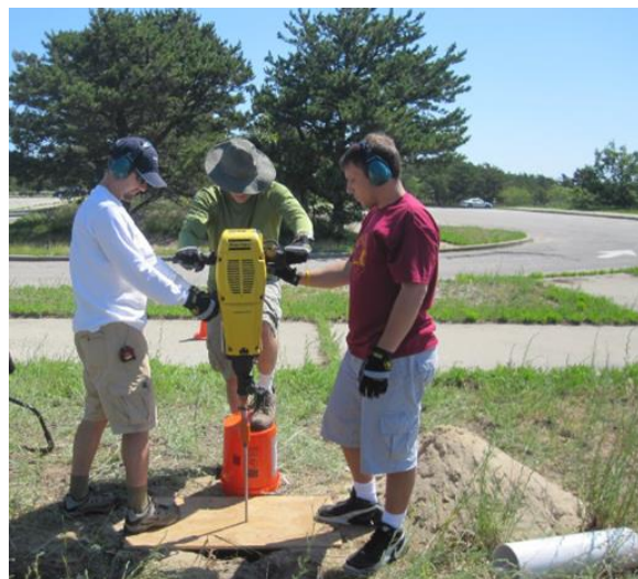
Fig. 40. Fig. 2. Using a gas powered jackhammer to drive the steel rods into the ground (from a URI guide for installing elevation monuments on National Park Lands).
