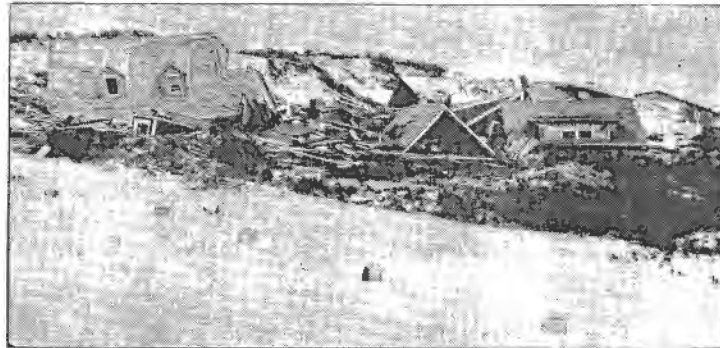
Houses jumbled like this at Horseneck's West Beach. The piles in the foreground once supported a residence.
