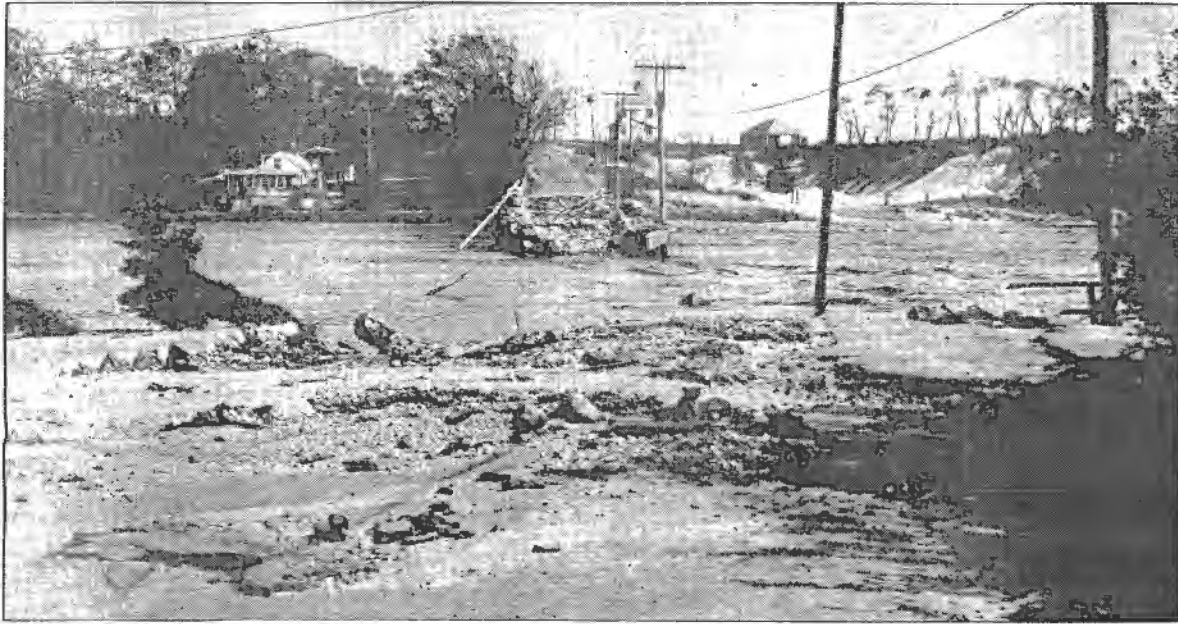
Hix Bridge was wiped out completely by the rushing waters. This picture, taken the day following the storm, shows nothing remaining except the bridge site.
