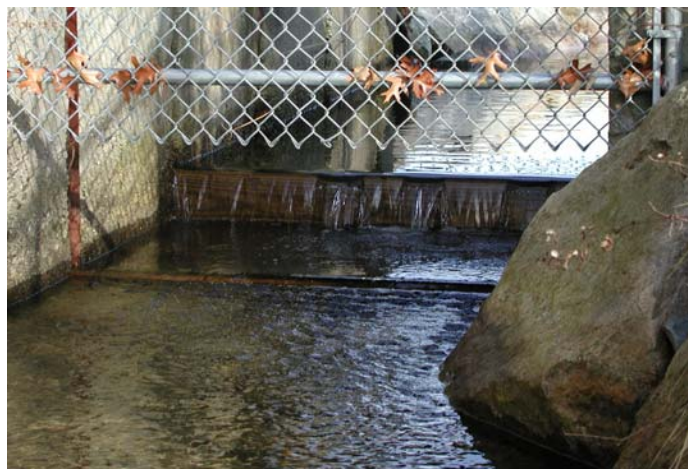
Fishway at Mashpee Pond Control Structure
