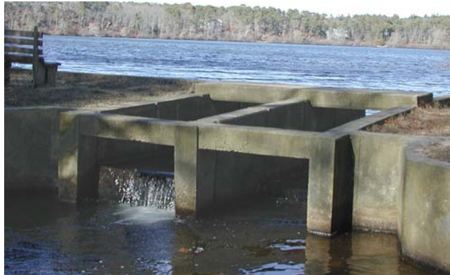
Hinckleys Pond Control Structure and Ladder
