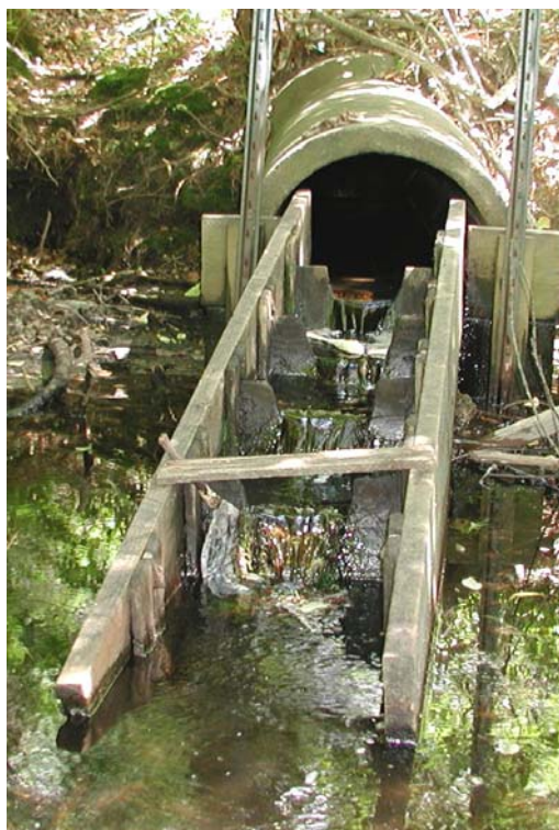
Clear Brook Road Culvert and Ladder
