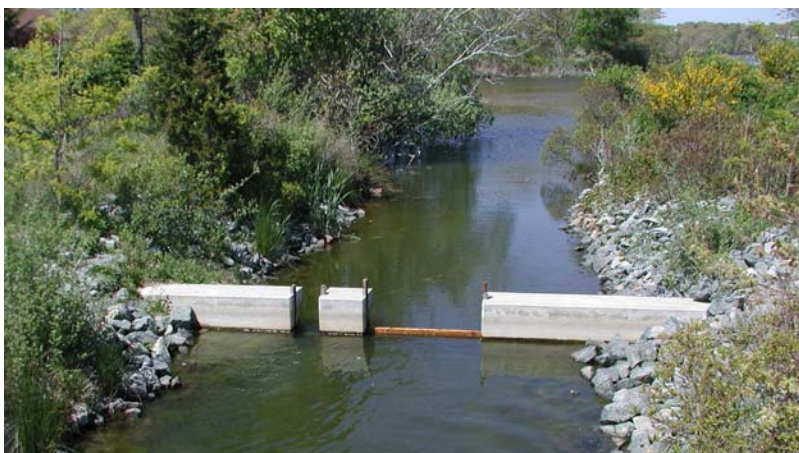
Oyster Pond control structure and fishway
