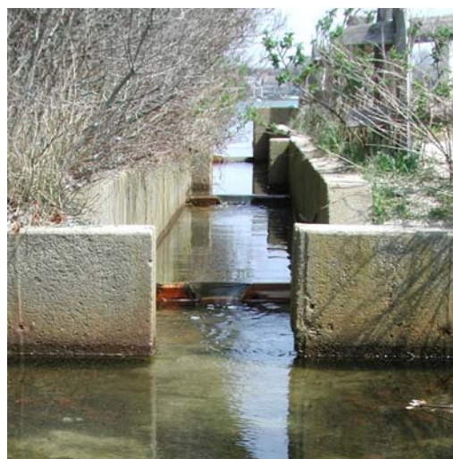
Notched Weir-pool at Herring Pond
