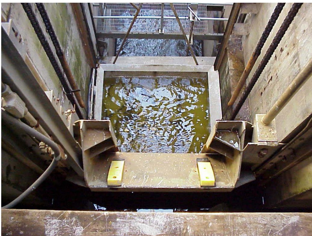
Fish lift – hopper rising with fish – Essex Dam, Lawrence
