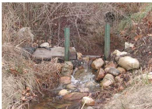
Fishway at John Parker Road culvert and bog sluice
