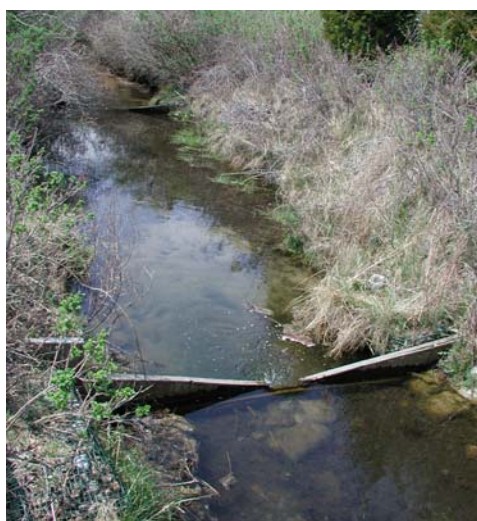
Herring Pond Stream Baffles
