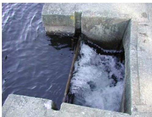
Spillway at West Reservoir Dam
