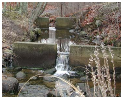
Stream baffles at Herring Brook Dam
