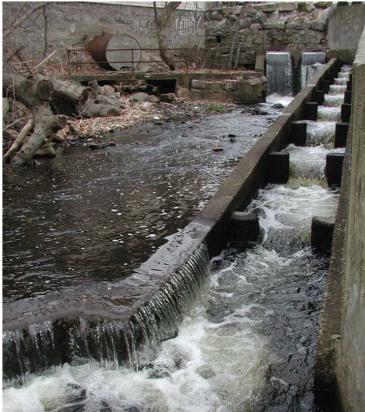
Notched weir pool fishway – Pleasant St. Dam, Weymouth
