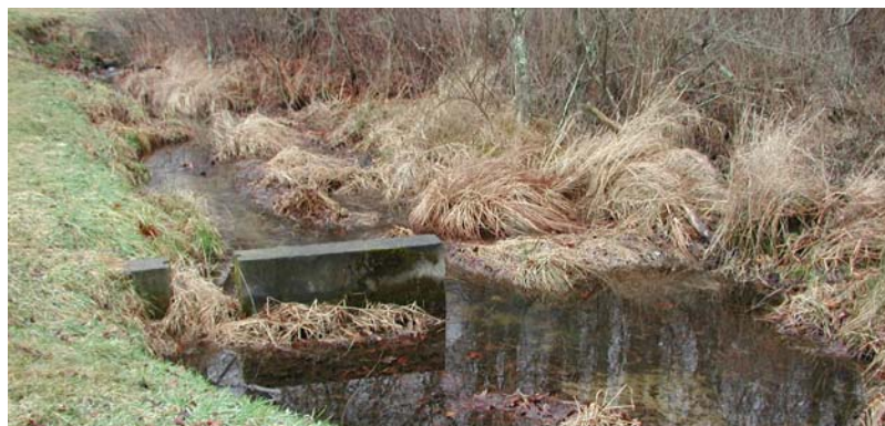
Bypassed stream baffles
