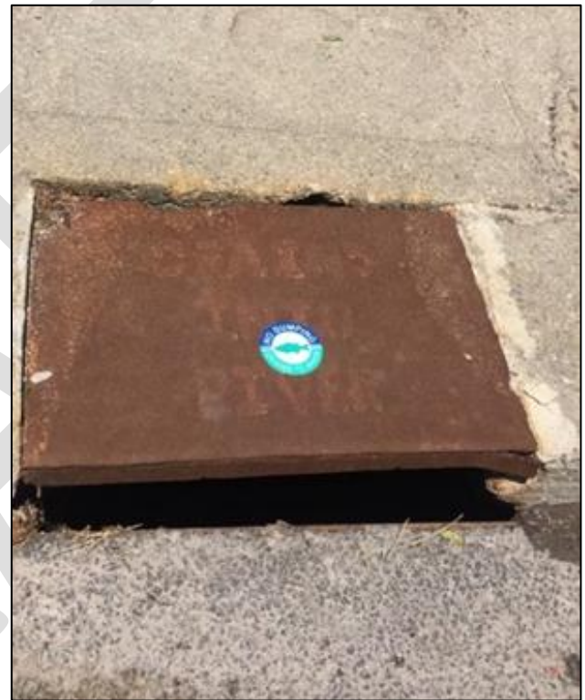
Figure 73. Open curb drain without grates may allow plastic bottles and other litter to enter storm drain networks.
