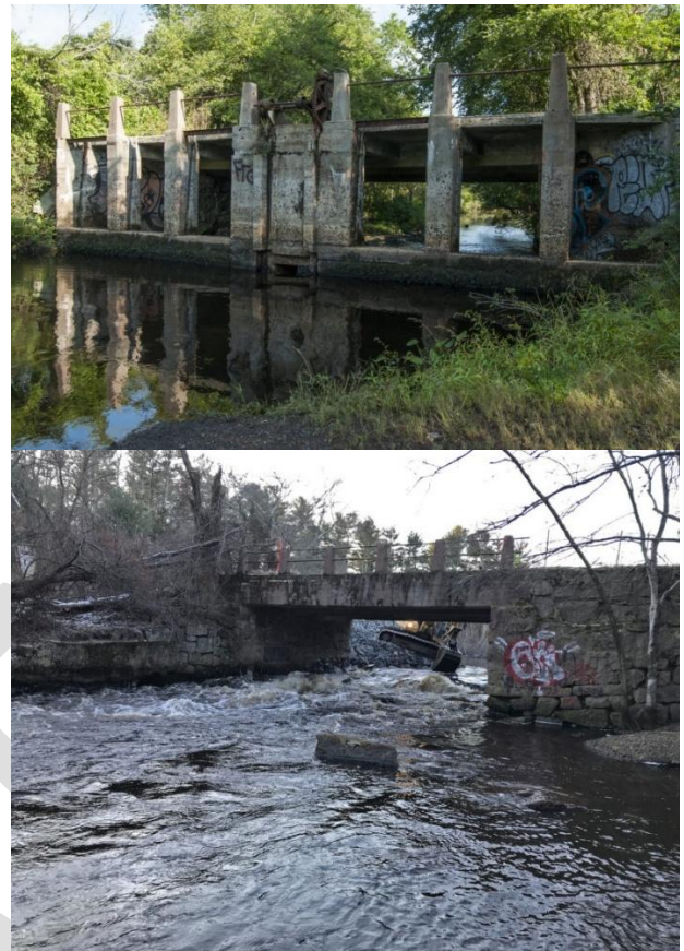
Figure 55. The Horseshoe Mill bridge before (top) and after (bottom) dam removal.
